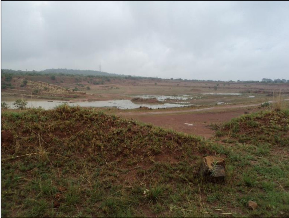
Figure 8: Main pit area.
