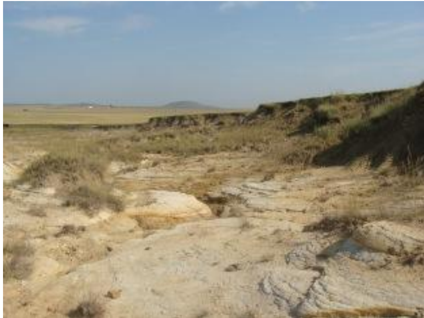
Figure 9: A closer view of one of the many erosion dongas/ drainage lines criss-crossing through the area.
