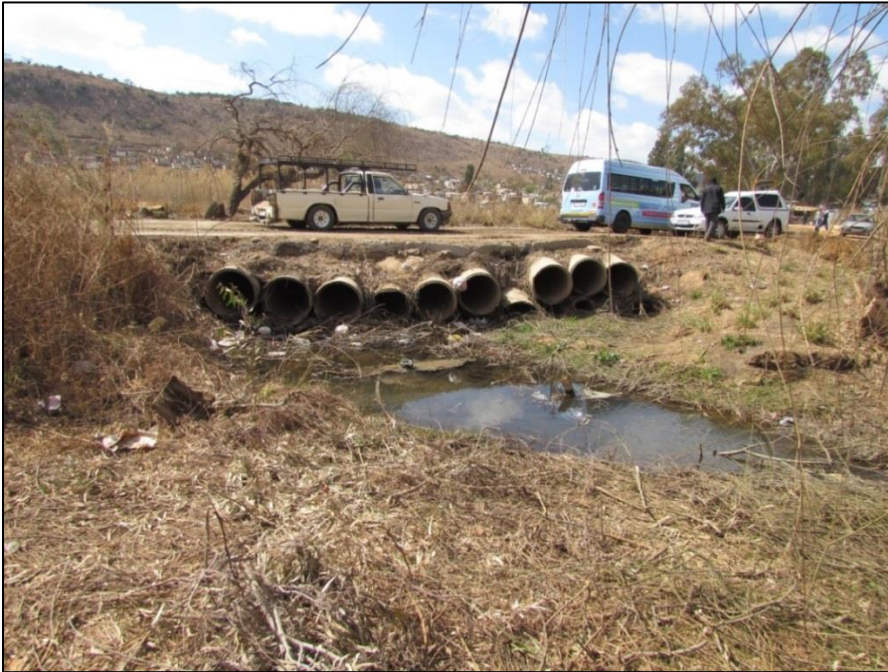
Figure 5-4: Existing Stoffel Park Project pipe bridge
