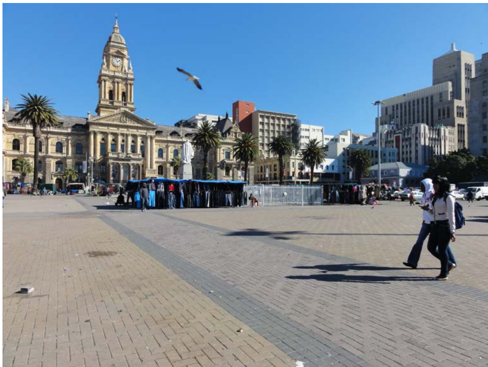
FIGURE 5: The current open space qualities of the Grand Parade: occasional traders, inappropriate service interventions and no clear directional movements. (Image: Attwell, October 2013).
