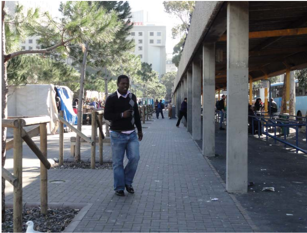
FIGURE 6: The Grand Parade edge of the Golden Arrow Bus Terminus which will be affected by the proposed stairway. (Image: Attwell, October 2013).
