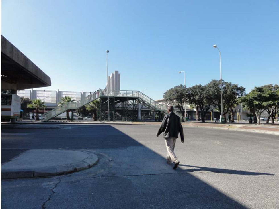
FIGURE 10: The current Strand Street pedestrian bridge showing the axial link with the Civic Centre. (Image: Attwell, October 2013).
