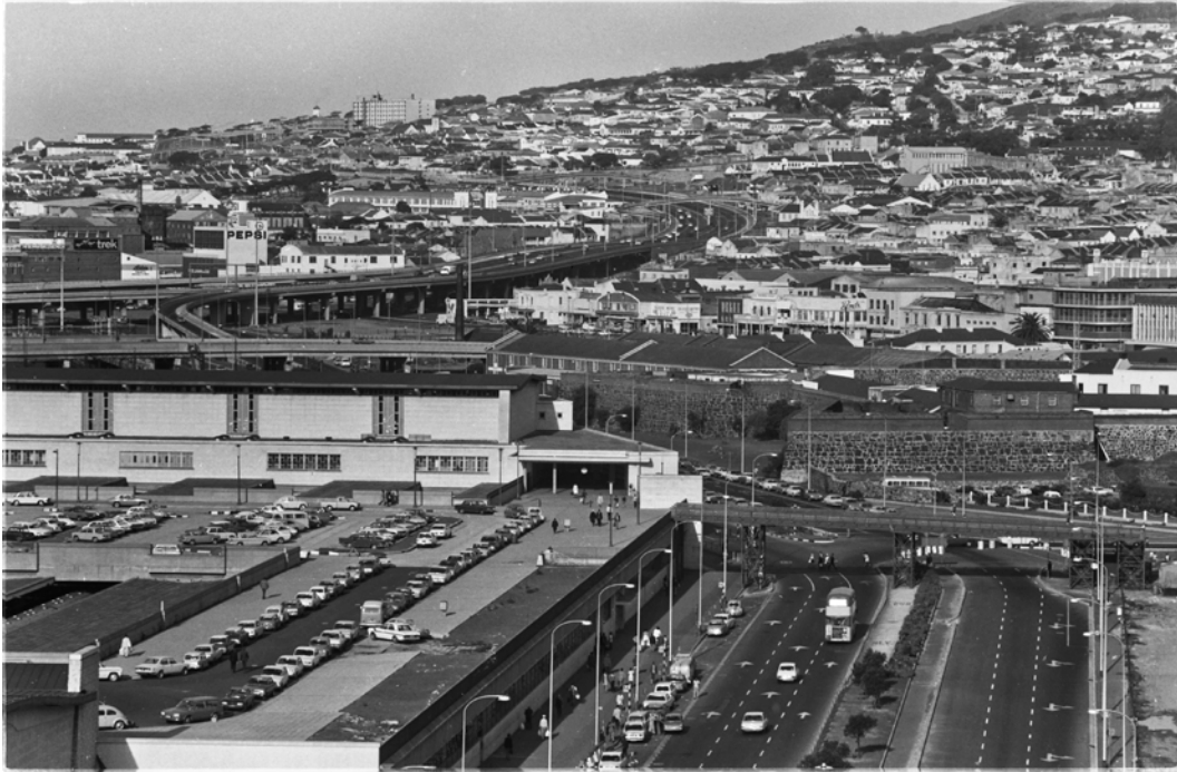
FIGURE 15: The Cape Town Station second or “non-white” concourse showing how the bridge was central to commuter access. City of Cape Town CCB135_f78-i2. The design carries through the use of overhangs, broad horizontal lines, sweeping roof lines, multi-textures and polychrome surfaces
