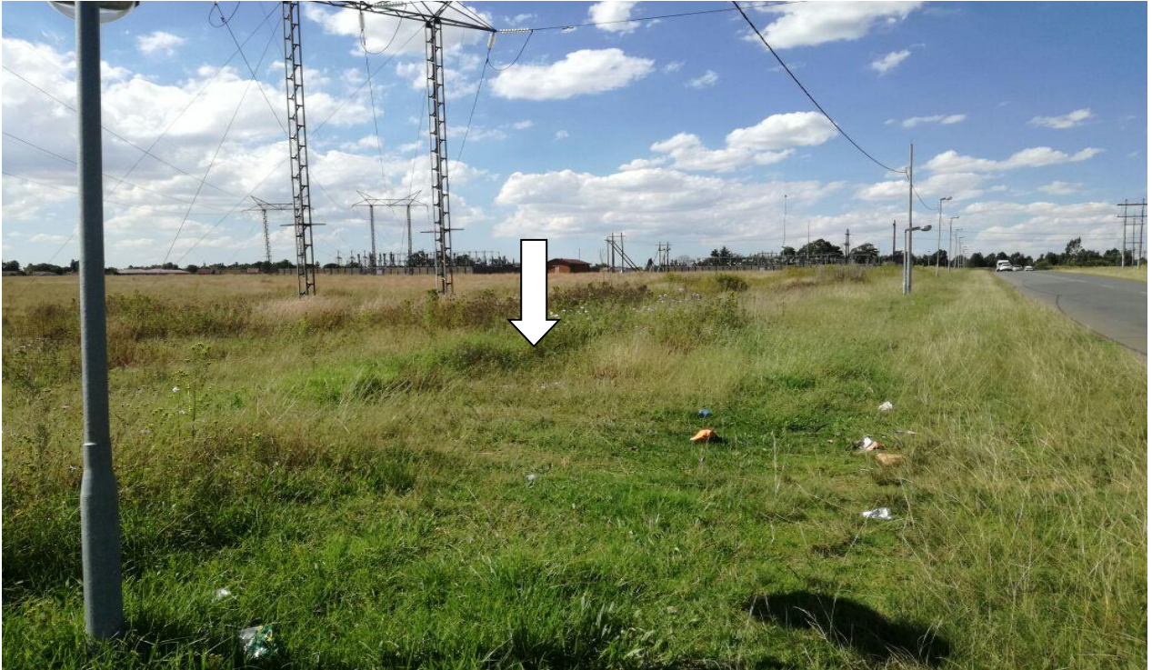
Plate 21: Shows terminal position between Eskom structures along the Cloverfield road servitude, Modder East Springs.
