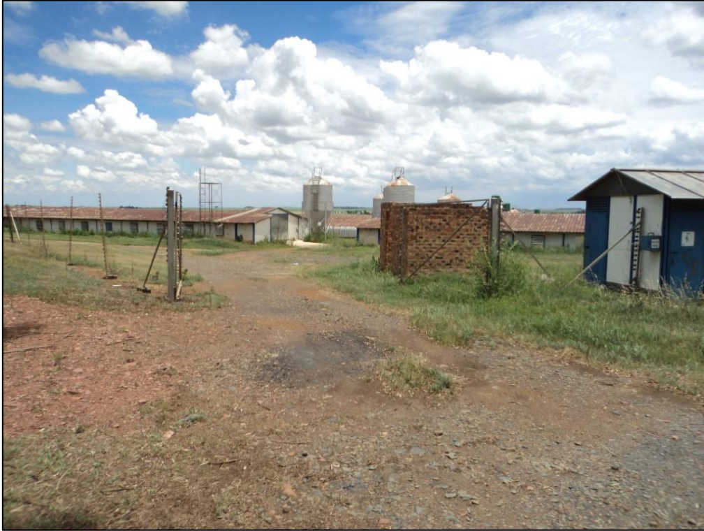
Figure 15: Entrance to the fenced-off infrastructure.
