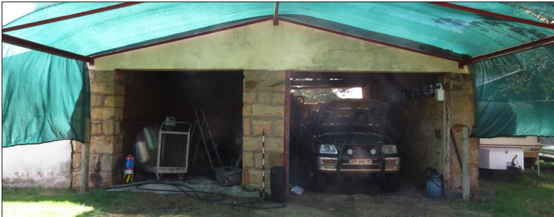
Figure 28 – General view of the structure.
