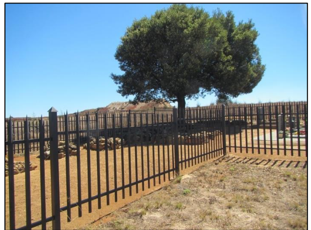
Figure 19 – Formal fence at ILM002
