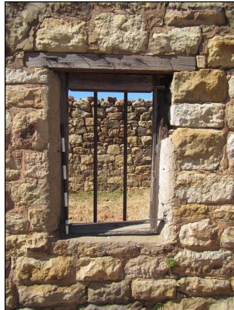
Figure 29 – View of barred windows at ILM007
