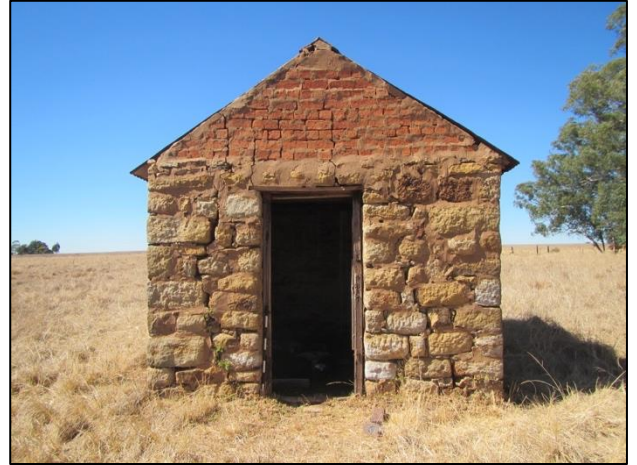
Figure 31 – Smaller shed behind the main structure (windows also barred)
