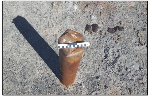
Figure 25 – Pipe has been sealed off
