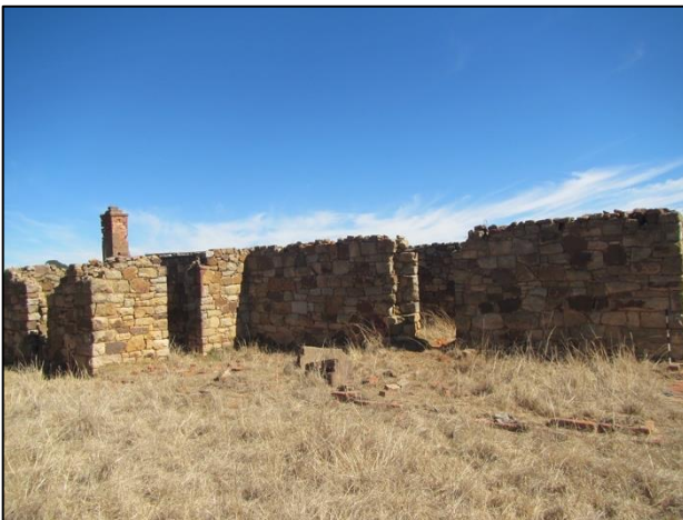
Figure 28 – General view of the main structure from behind.
