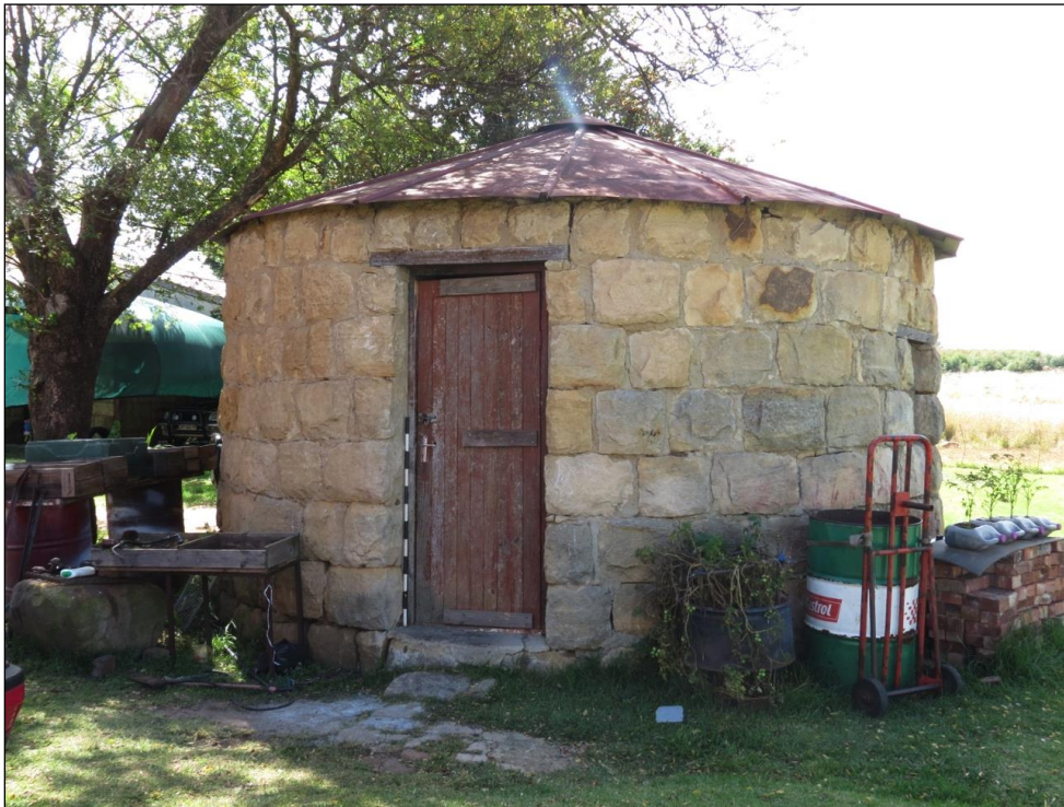
Figure 26 – General view of the rondavel structure. Note the lintel, door and doorframe all manufactured of wood.
