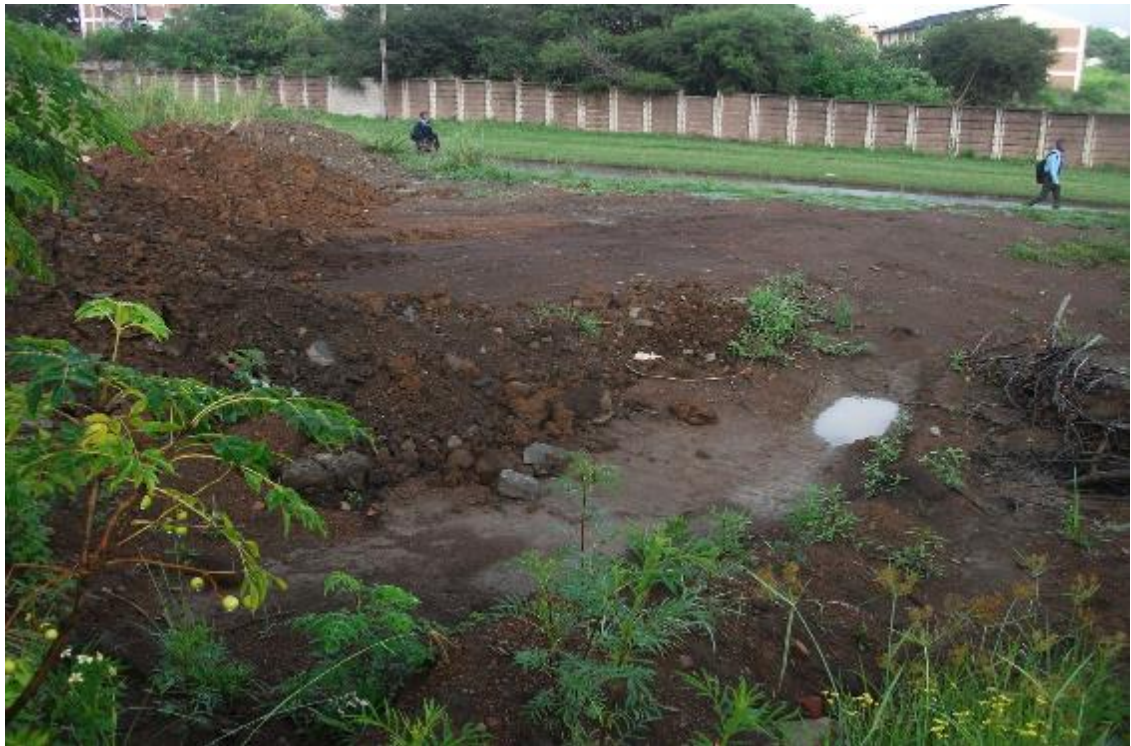
Figure 6: Removal of soil from site near road
