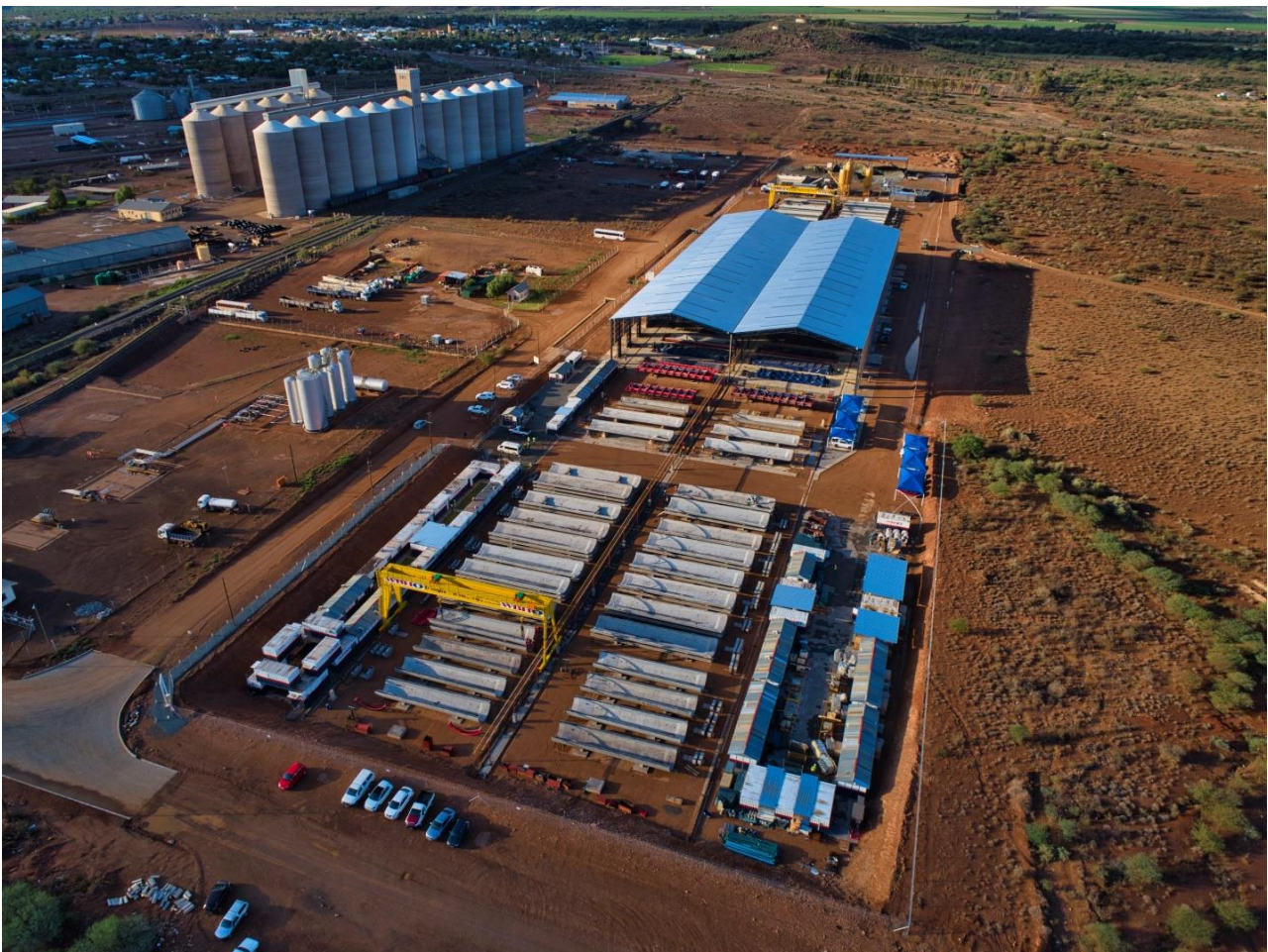
Figure 4: Typical site layout (aerial image of the factory).
