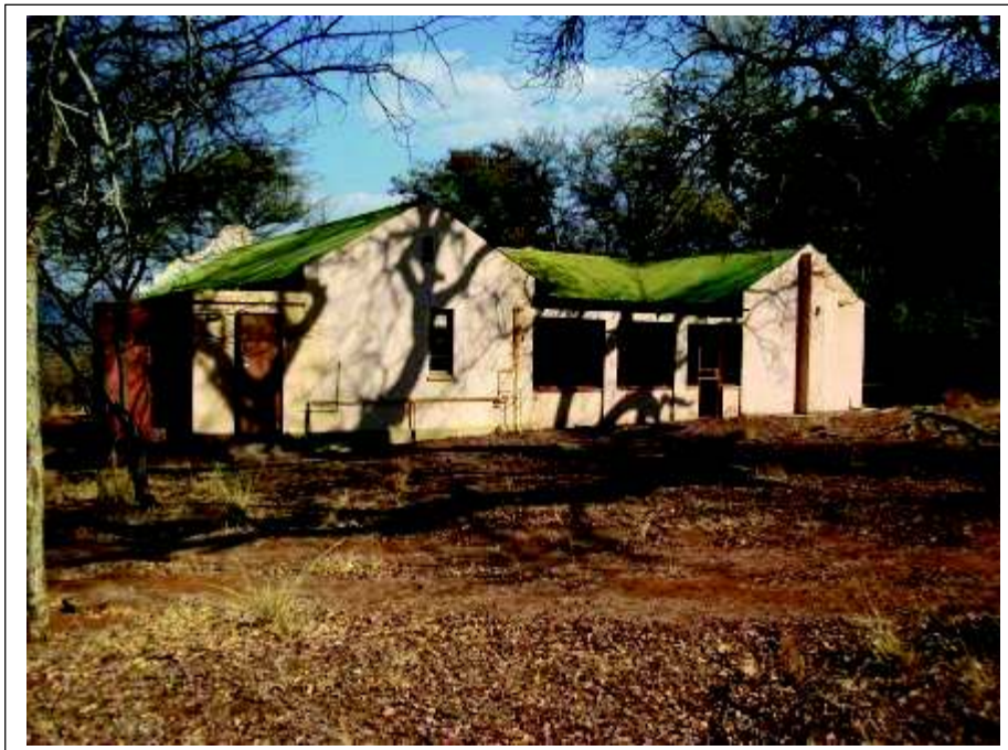
Figure 36- Back view of historical residence on Randstephne 455KQ (above).
