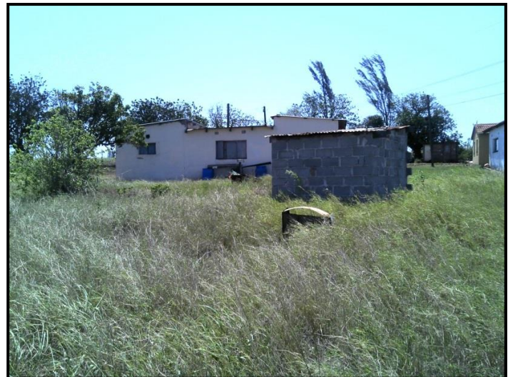
Figure 16. Outbuildings at feature 6.
