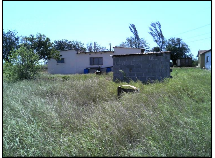
Figure 17. Outbuildings at feature 6.
