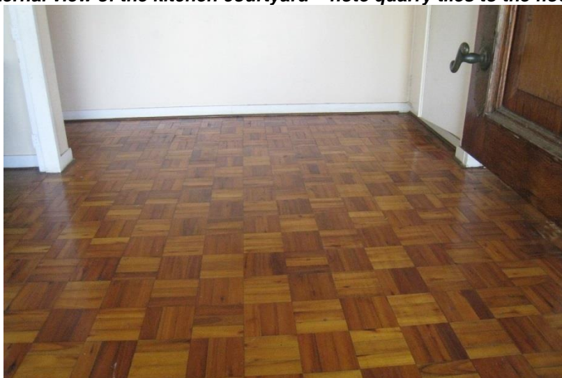
Fig 57: Internal view of reception rooms with parquet flooring
