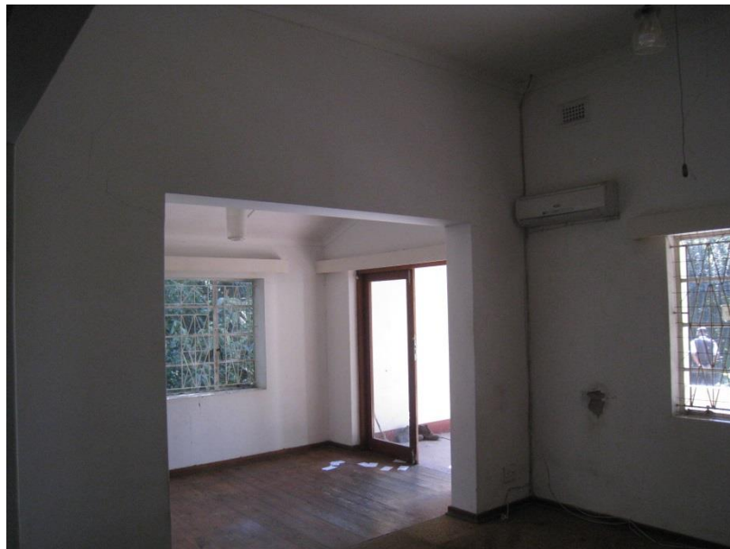
Fig 29: Access onto veranda, reception rooms
