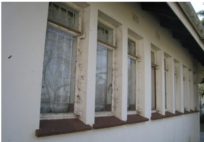
Fig 53: Row of windows to the east elevation
