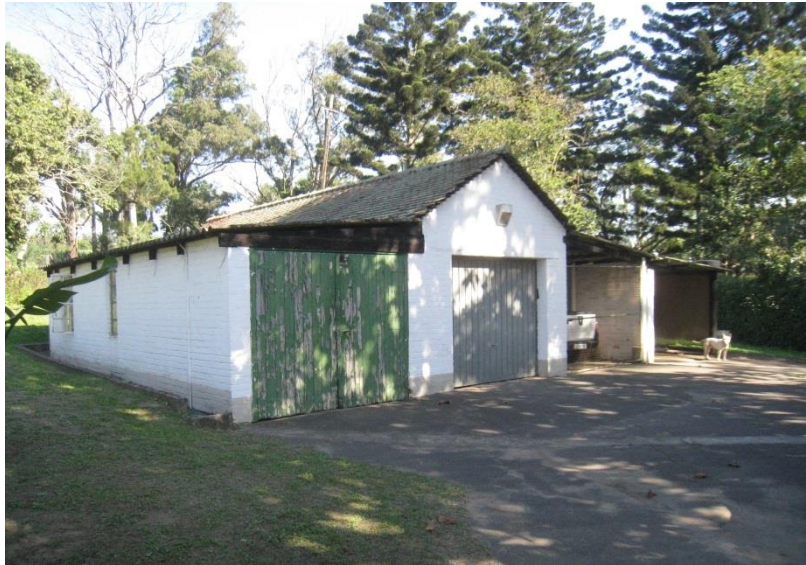
Fig 19: Outbuilding at House 1, showing accretions to both long sides
