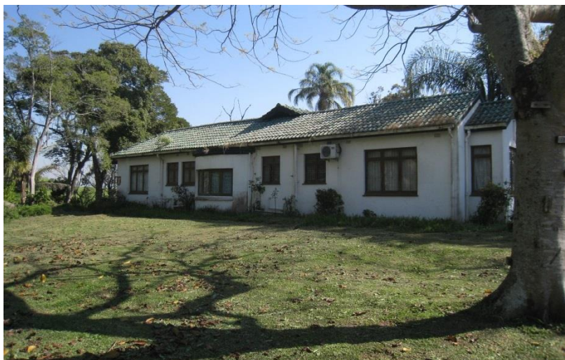
Fig 64: Eastern elevation, showing form of roof and green ceramic roof tiles
