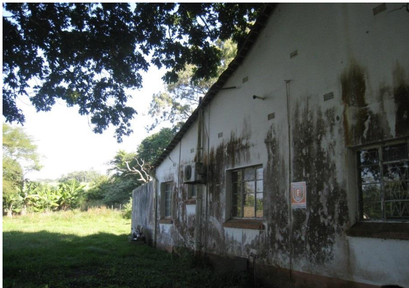
Fig 40: View towards the south of the east elevation
