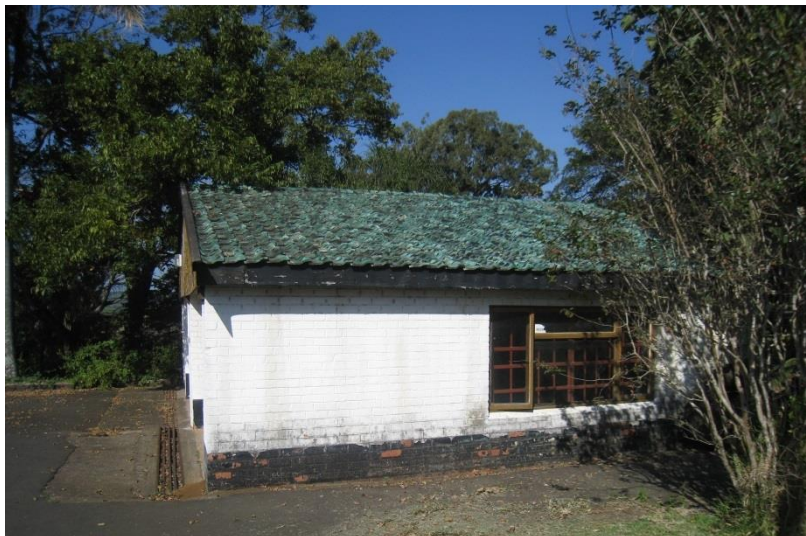
Fig 61: View of garage roof
