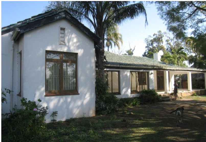
Fig 63: Main elevation, roughly north, showing deep veranda entertainment space
