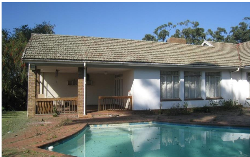
Fig 51: Looking into stoep / entertainment area
