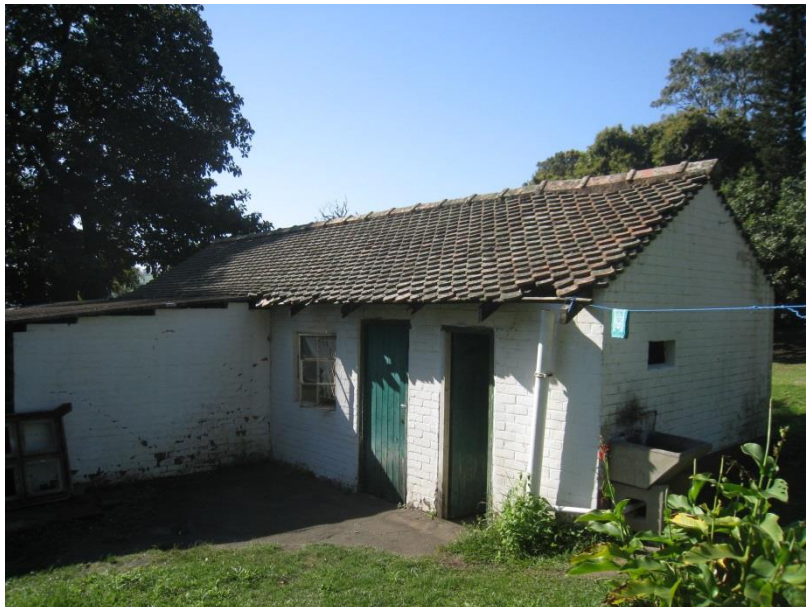
Fig 16: Rear elevation of Outbuilding, House 1
