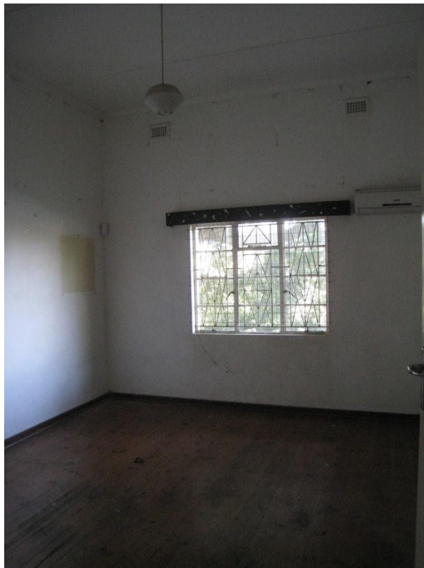
Fig 31: Bedroom facing east
