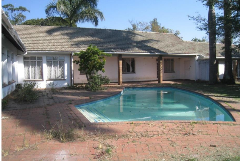
Fig 49: General view of the north facing elevation, around the entertainment area
