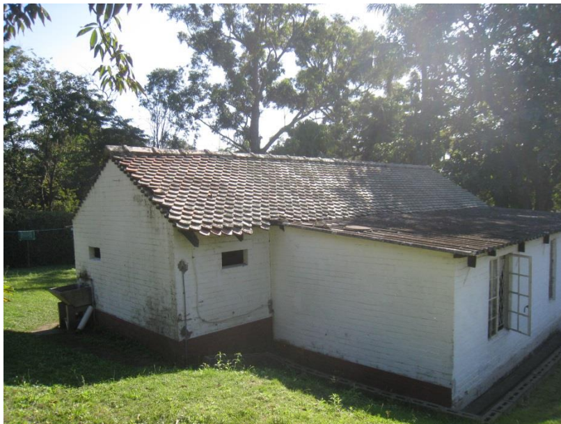
Fig 18: Outbuilding of House 1, showing main roof tiled in Broseley tiles
