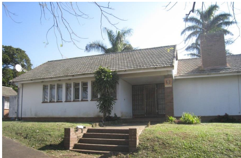
Fig 47: View of house from driveway, looking at entrance porch
