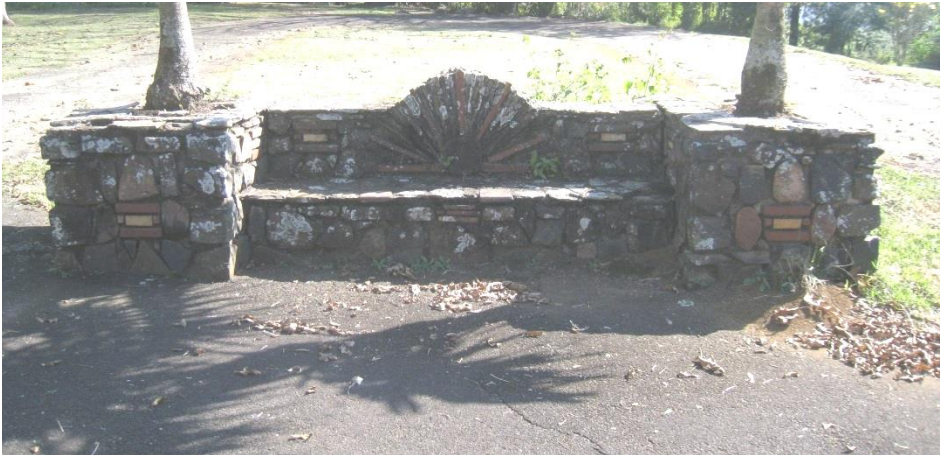
Love seat at the top of the driveway, no 6 Hospital Road
