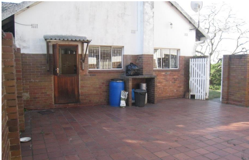
Fig 56: Internal view of the kitchen courtyard – note quarry tiles to the floor
