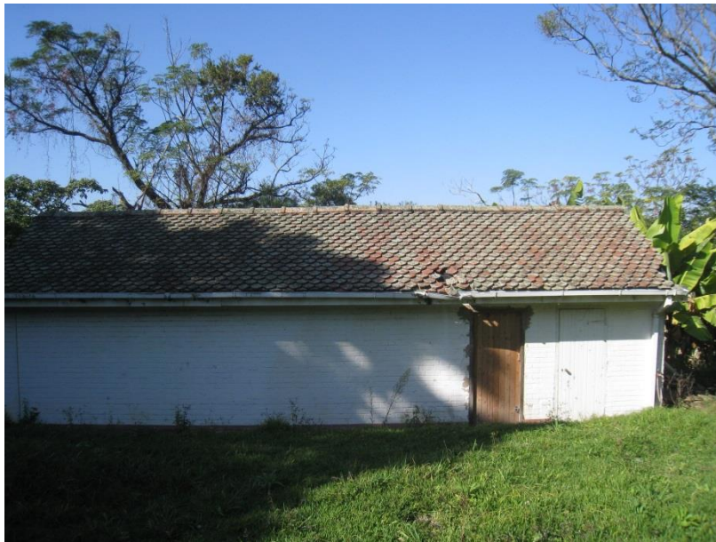
Fig 43: Outbuilding to House 3 – note Broseley tiled roof
