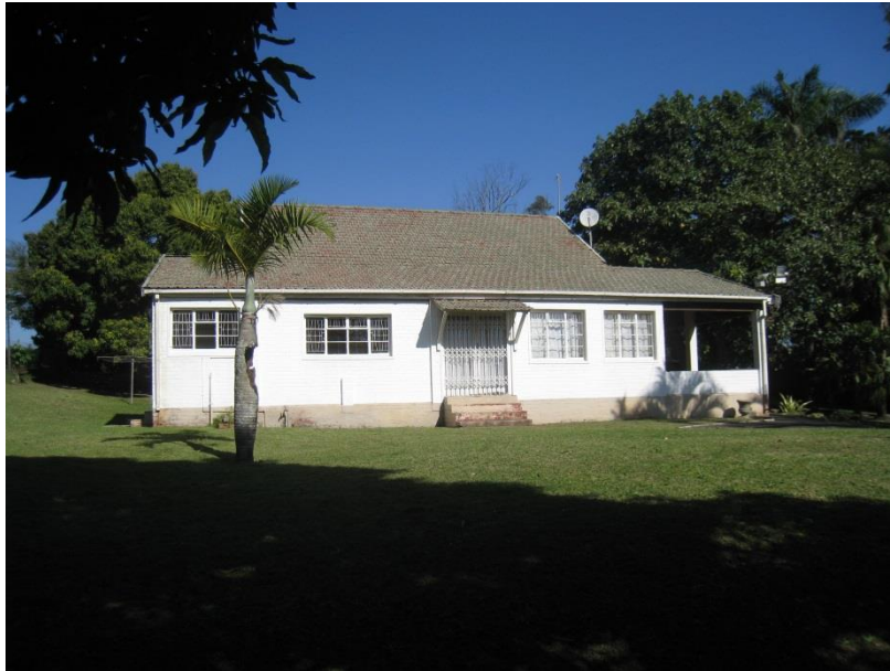
Fig 15: Elevation roughly facing north
