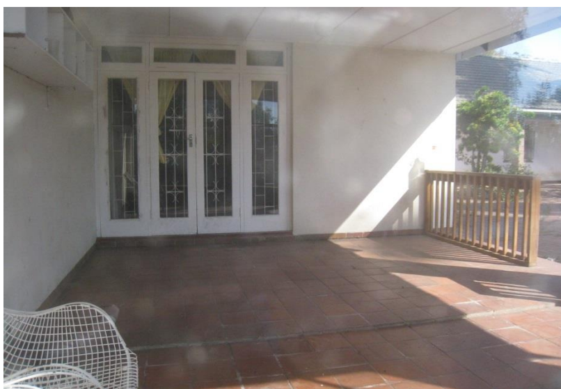
Fig 48: View of stoep (on the north-west), 4 Hospital Hill
