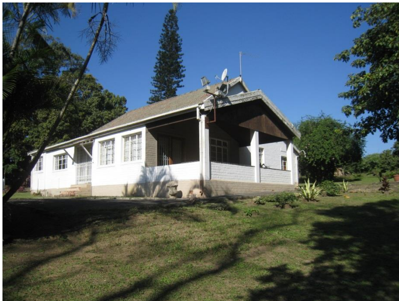
Fig 12: House Number 1 from the north-east corner
