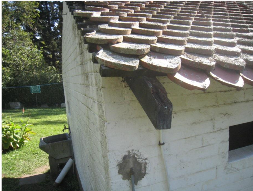
Fig 17: Detail of Broseley tiles to outbuilding at House 1
