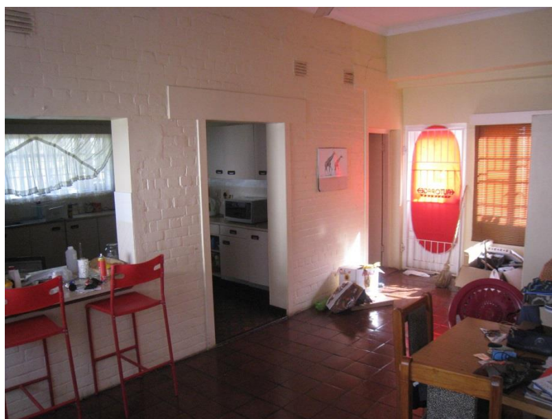
Fig 67: Internal view showing quarry tiled floor
