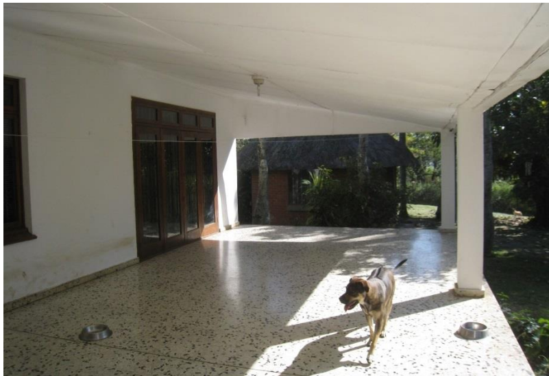
Fig 66: Terrazzo finished veranda
