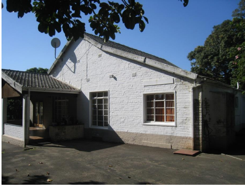
Fig 13: View of main house from the north-west corner
