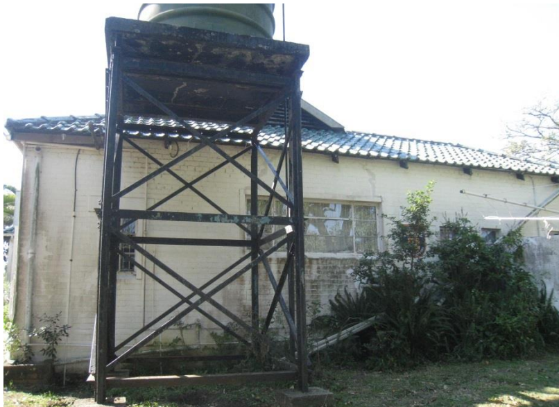
Fig 71: South-western corner with water tank
