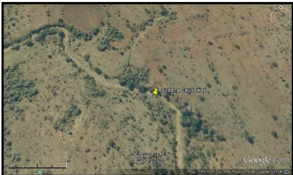
Figure 2. Google aerial photograph showing the road adjacent to the proposed Isdudana Causeway.
