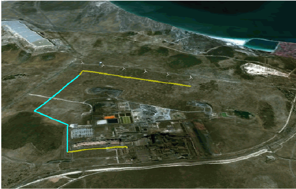
Figure 2. Simulated oblique aerial view of the site, looking south. Underground cabling trenches shown in yellow, overhead connection shown in cyan. From Google Earth.
