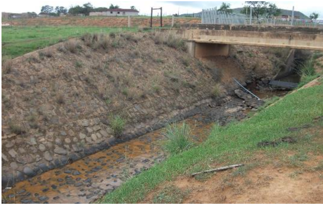
Figure 4: Canal / storm water drain
