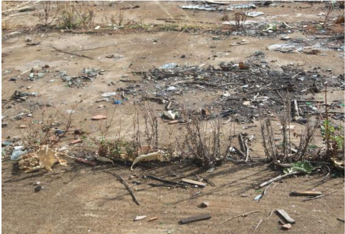
Figure 3: Remains of concrete floor
