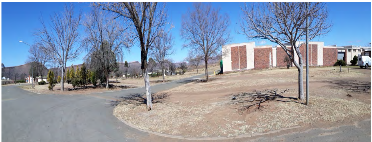
Figure 2. General view of existing prison facility located in Area 1, looking east (top), southeast (center) and south (bottom).
