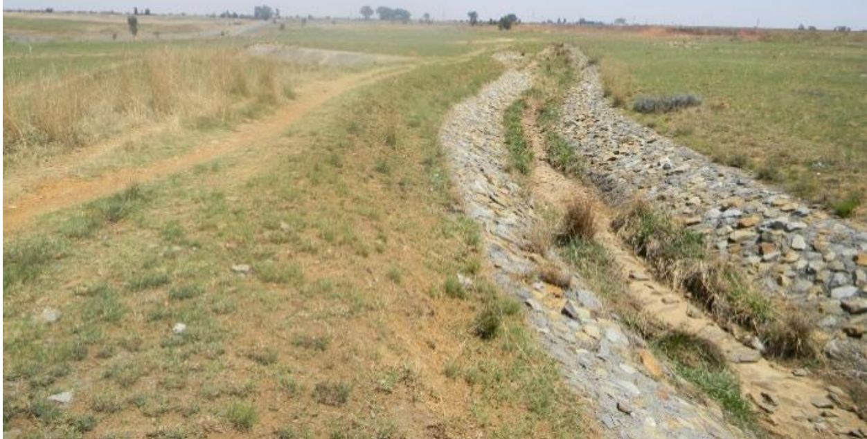
Plate 11: Photo K. showing the erosion control along proposed powerline route.
