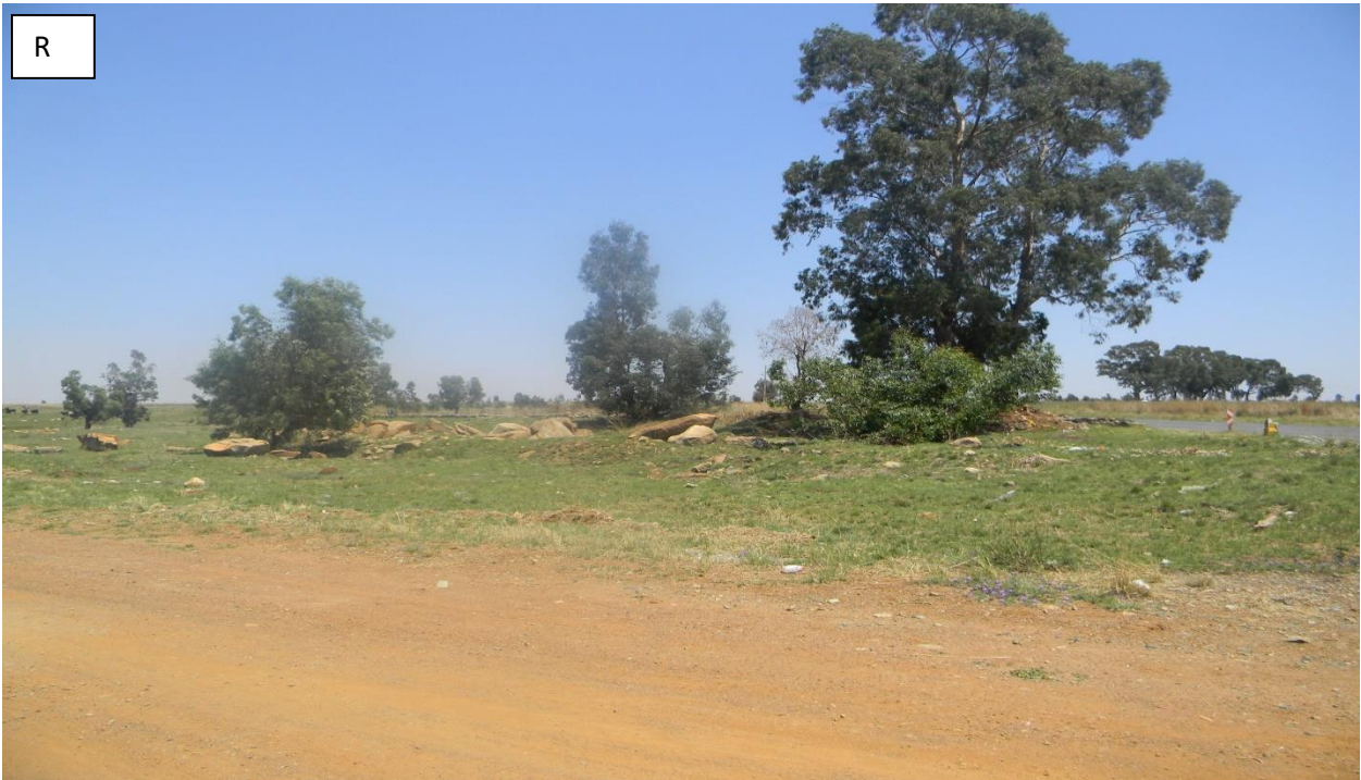
Plate 18: Photo R showing old sewer pipeline earmarked for replacement
