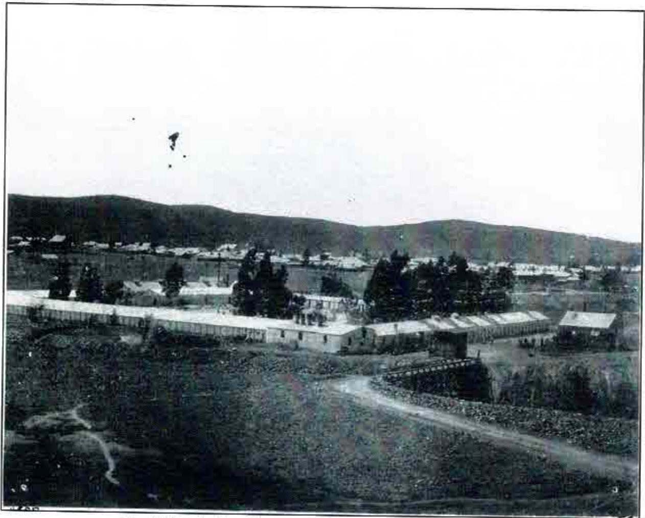
Figure 16. An early picture of the workers compound
