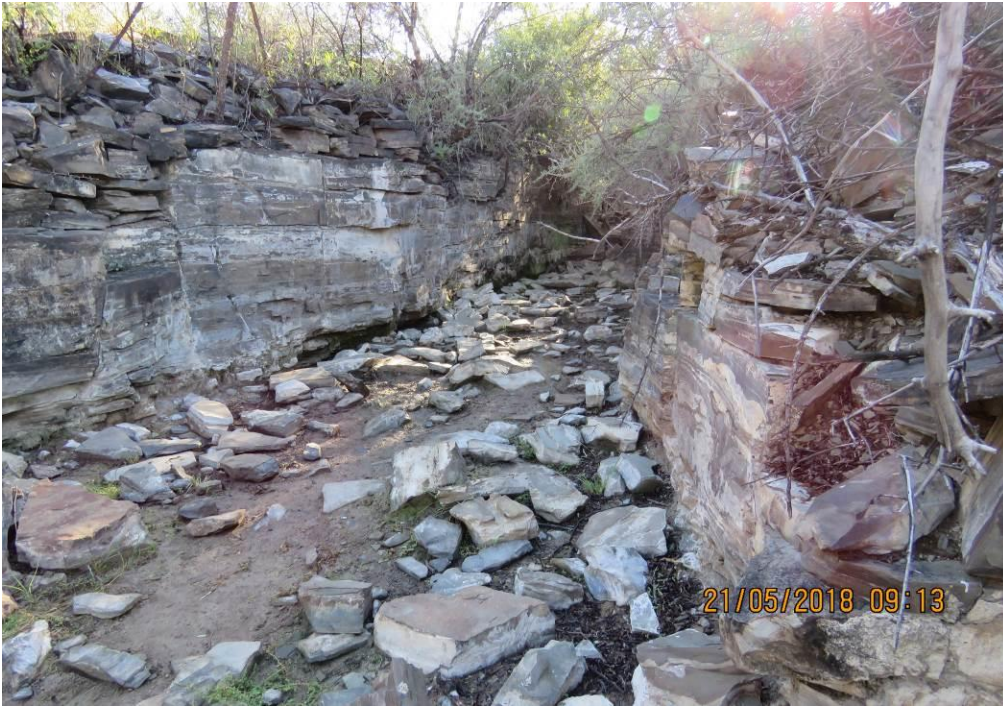
Figure 17. Spring source enlarged by cutting into the hill-side. (Adjacent to observations 7 and 8).
