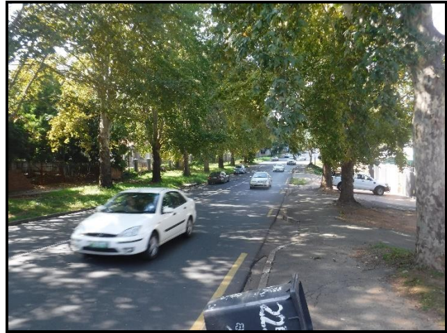
Figure 10: General site conditions.
