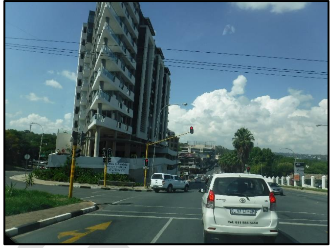
Figure 7. General Site conditions
