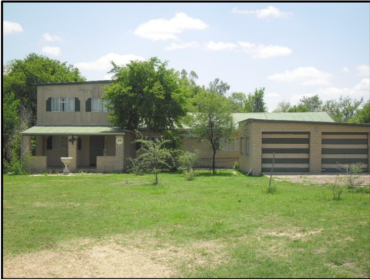
Figure 7. Existing building on site.
