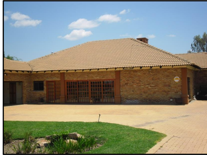
Figure 6. Existing building on site.
