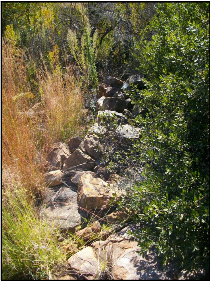
Figure 23: Stone walling at Site 4
