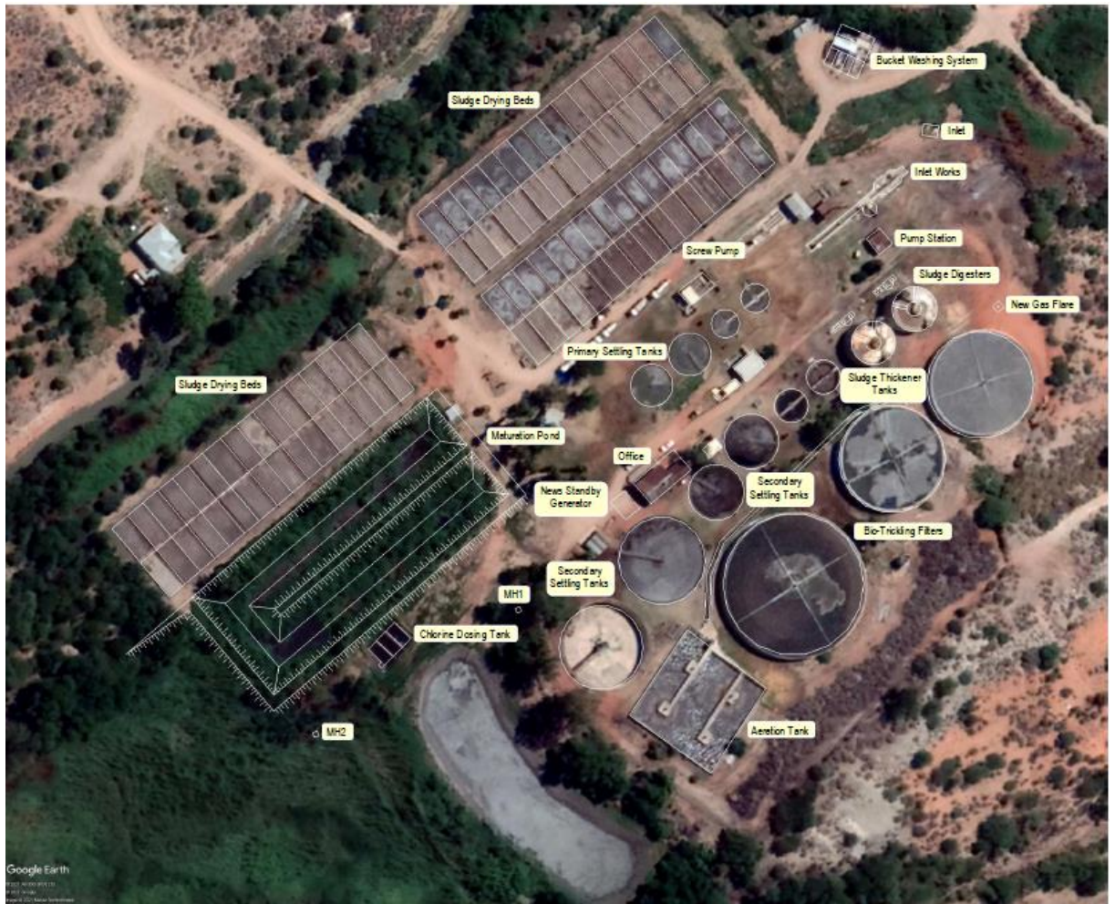
Figure 3: K-WWTW existing infrastructure to be refurbished (Google Earth image as supplied by the developer).
