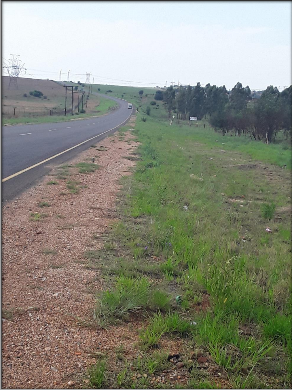
Figure 14: End of proposed road construction. No fossiliferous outcrops are present. GPS Coordinates 25°54'30.57"S 28°19'29.39"E
