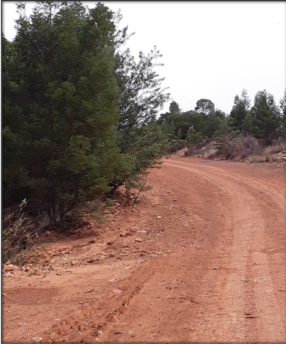
Figure 9: Big trees present in the proposed development. No fossiliferous outcrops are present. GPS Coordinates 25°51'8.17"S 28°20'52.96"E
