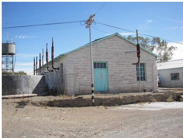
Figure 43: Old Power Station.
