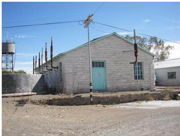
Figure 44: Old Power Station.
