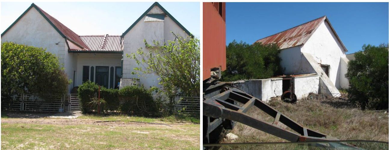
Figure 3 Vaatjie main house (left) and outbuilding (right).
