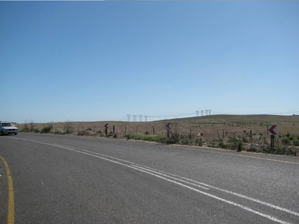
Figure 3 Above: view of existing 400 kV transmission lines from the turnoff to Oliphants Kop Farm.
