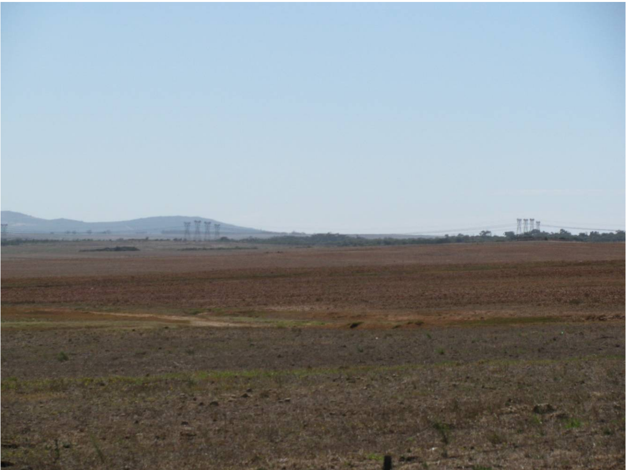
Figure 2 4x400 kV transmission lines Koeberg – Omega viewed from roughly 2000 m in open landscape.
