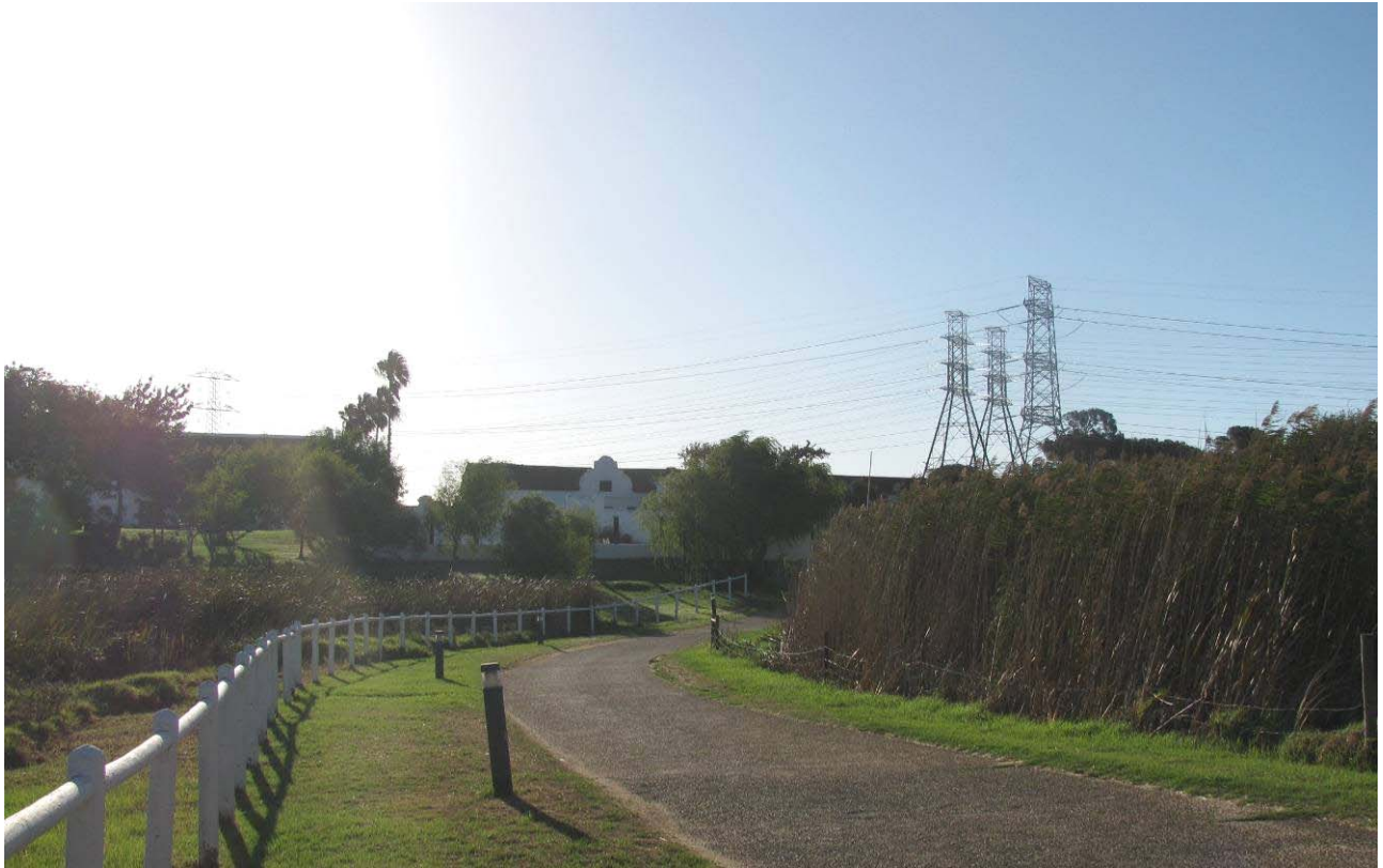
Figure 4 Transmission lines and towers located some 80 m behind the farm buildings at Hazendal Provincial Heritage Site dominate the view towards the buildings and destroy the sense of history of the place.
