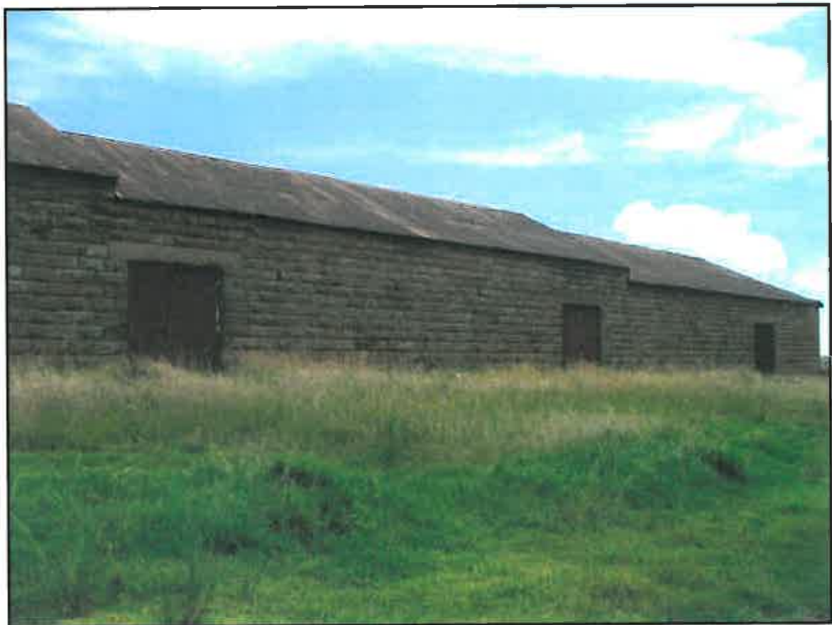
• Figure 23 – View of structure
