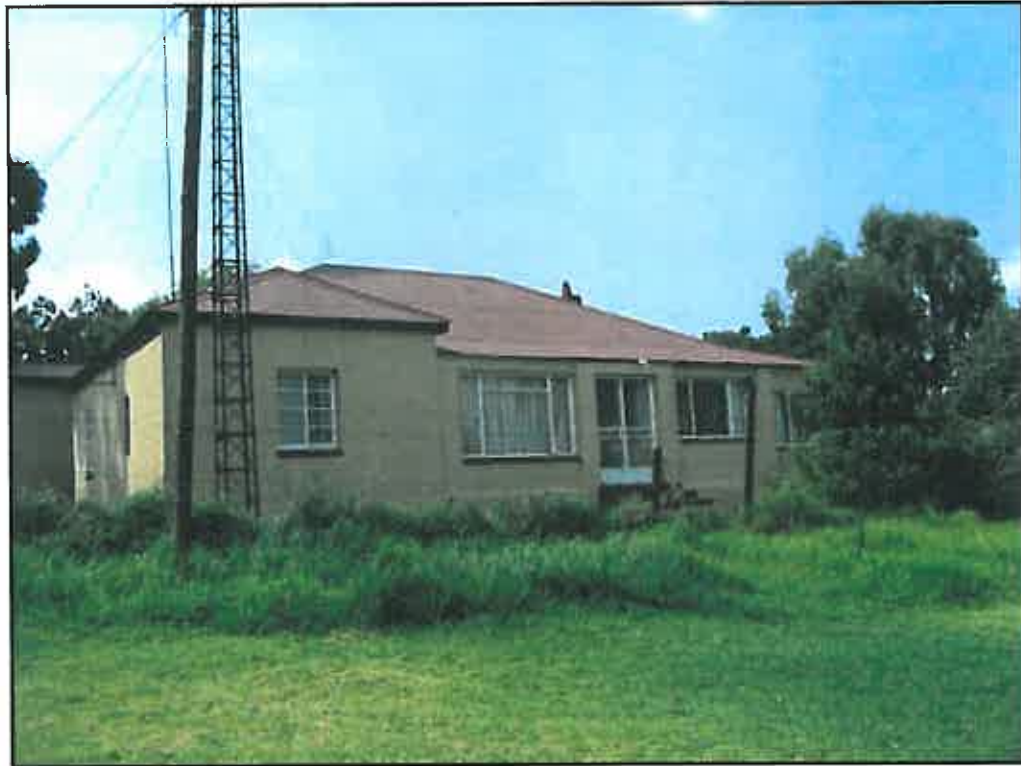
• Figure 17 – Main house
