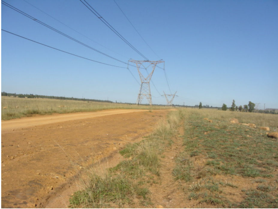
Figure 9: Power lines running across the surveyed area.
