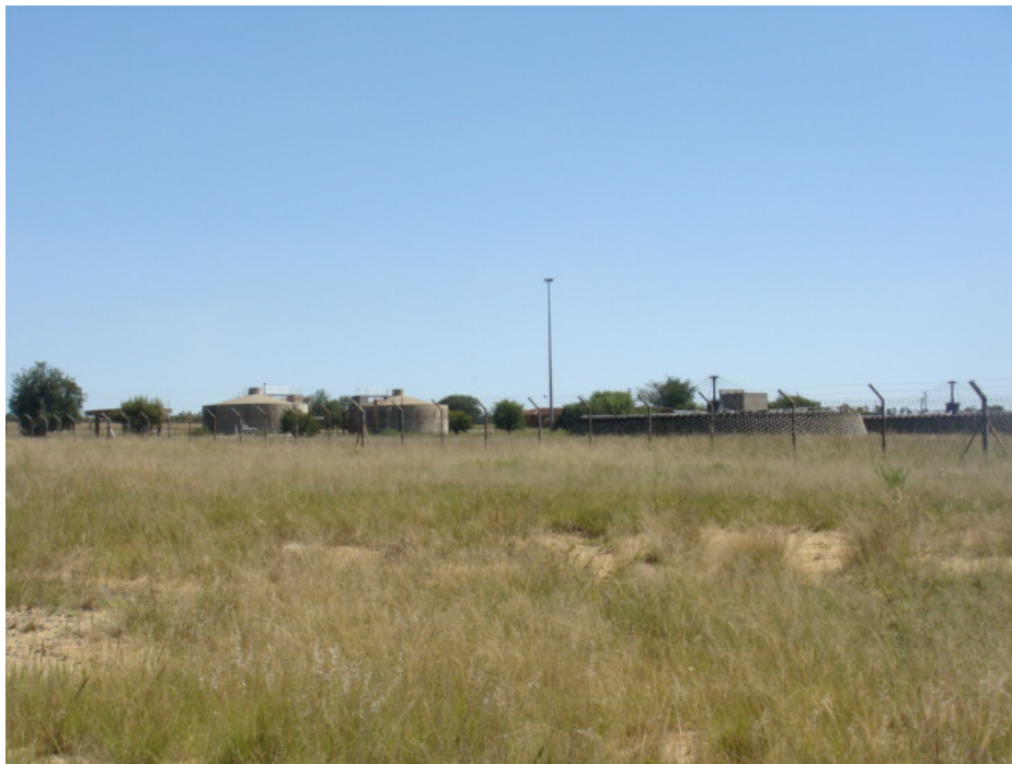
Figure 17: The existing Klipspruit Sewage Treatment Works.
