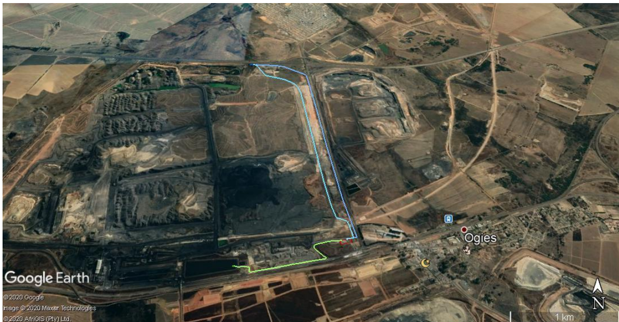
Figure 1: Google Earth map indicating the pipeline route for the Klipspruit WTP. Note the extensive alteration of the whole area.
