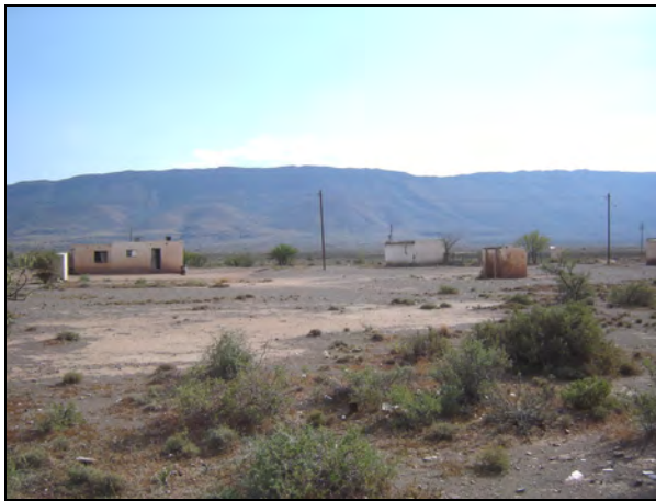
Former labourer's cottages
