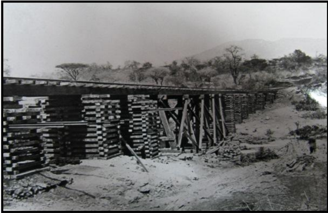
Fig. 4.7. A bridge at Kaapmuiden constructed by the Six Companies of the Brigade of Guards within two days during the ABO (1899-1902; no date).
