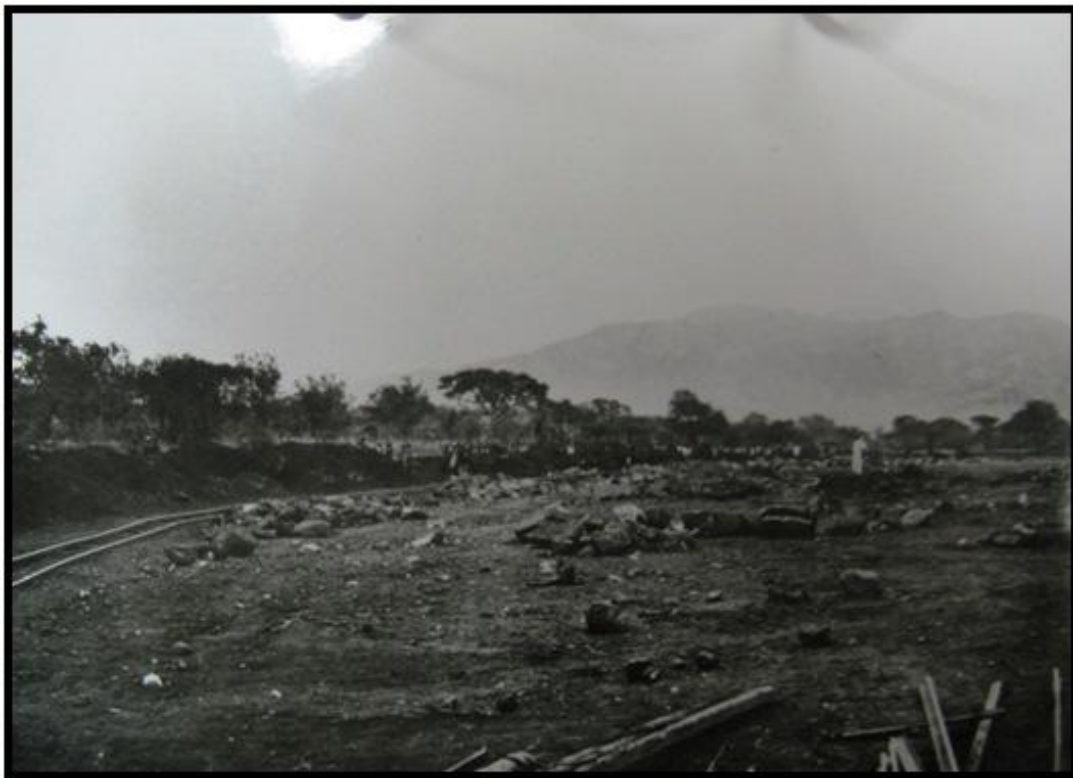
Fig. 4.4. The construction of the Delagoa Bay railway line in the vicinity of Kaapmuiden.
