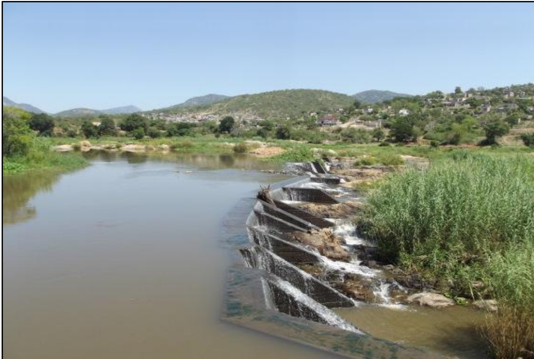
Fig. 30. Site KP 23. The weir in the Crocodile River. Photo taken in north-western direction.
