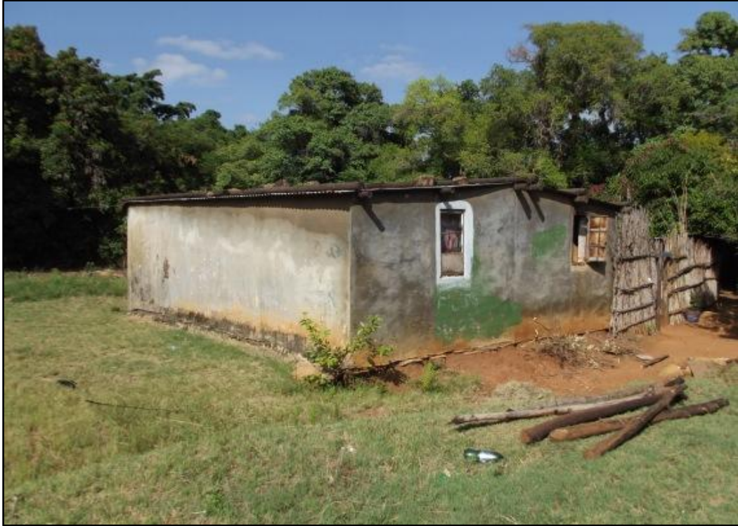
Fig. 3. Site KP 2. Farm worker's house. Photo taken in south-western direction.
