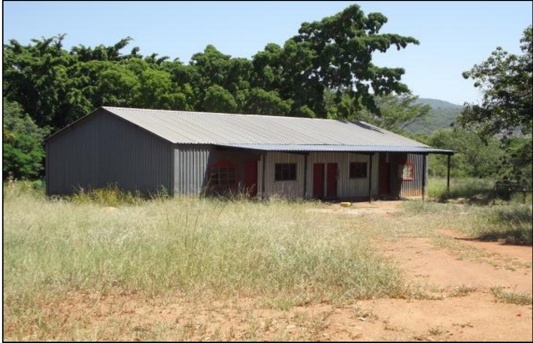
Fig. 13. Site KP 12. Farm shed. Photo taken in north-western direction.
