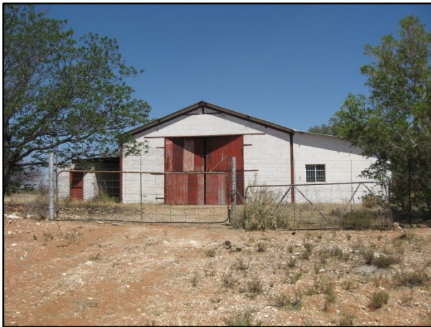
Figure 11 - View of the brick-built structure from the east
