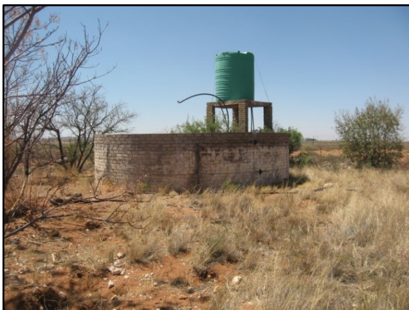
Figure 12 - View of the cement dam in the yard
