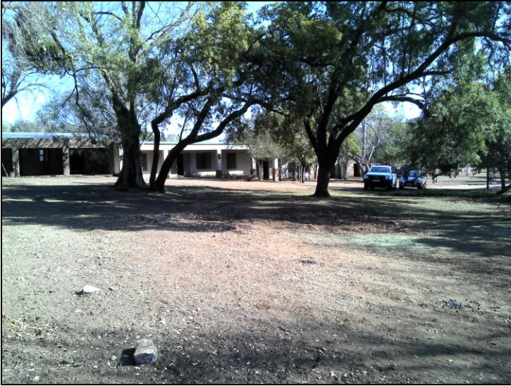
Figure 4: General site conditions.
