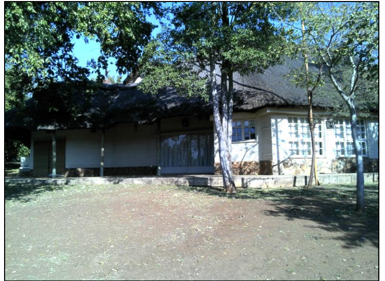
Figure 7: General site conditions.
