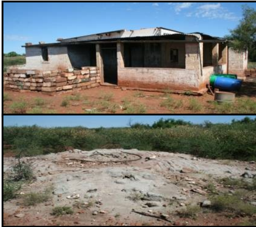
FIG. 6: HOUSE AND ERODED MUD BRICK FEATURE
