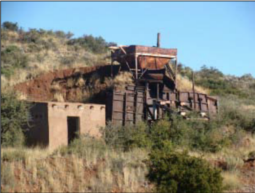
Figure 21. Ore Crushing Facility (Van Vollenhoven 2009)
