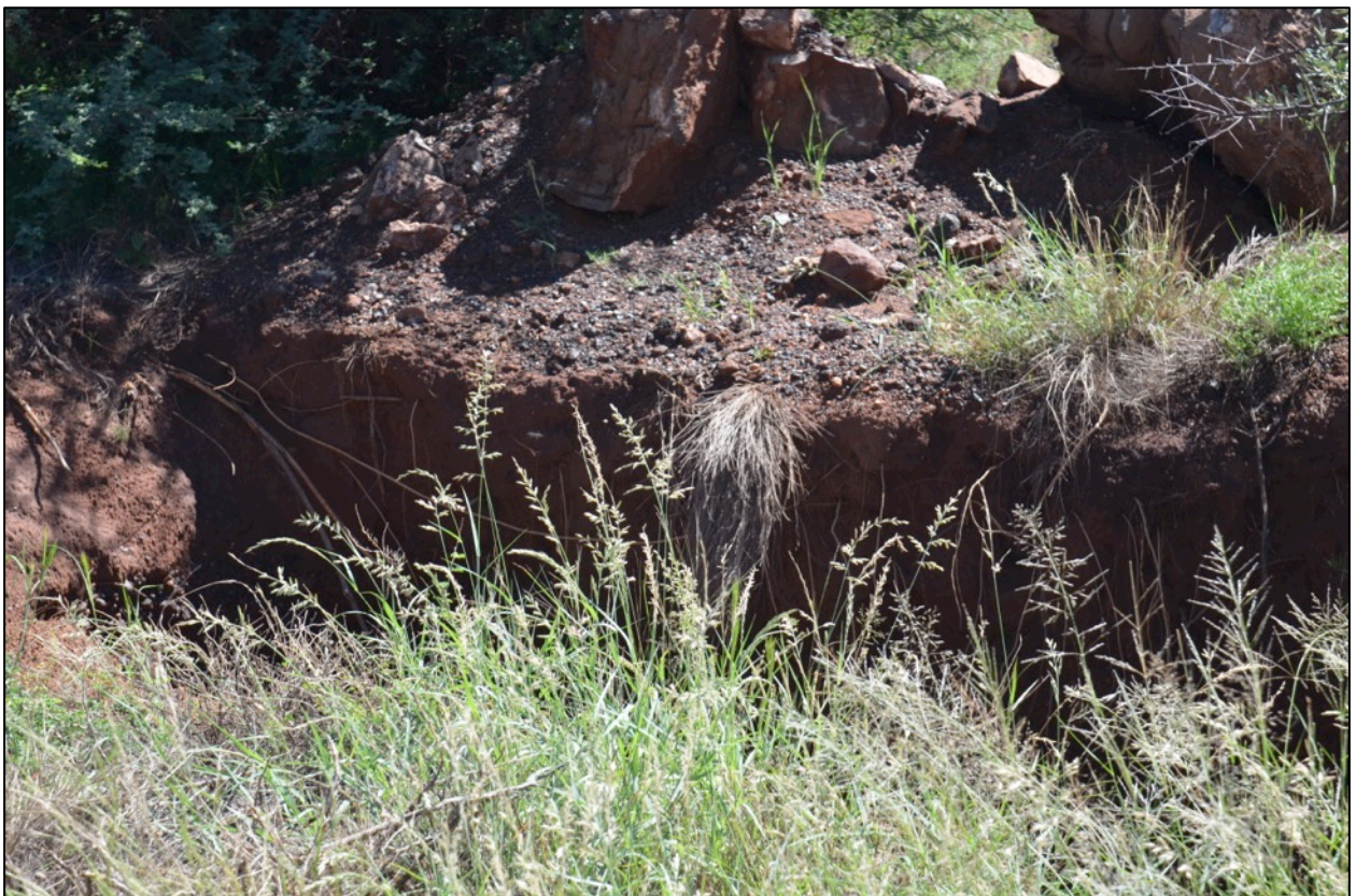
Figure 3. Geotechnical excavations showing magnetite rocks
