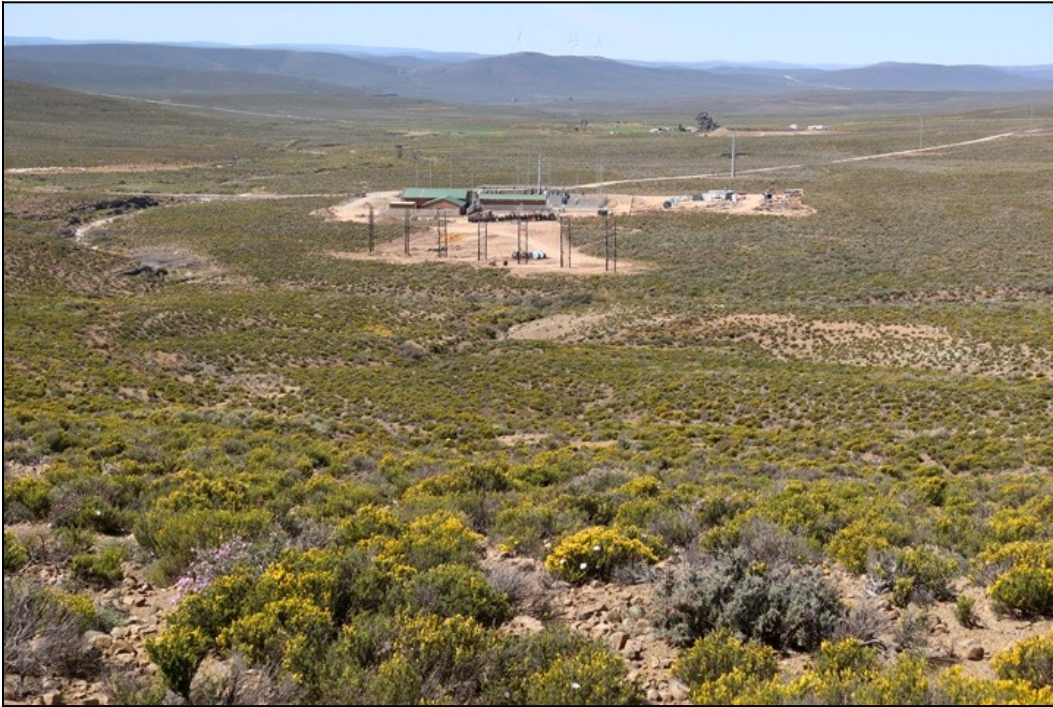
Figure 6: View from the SW towards the new Eskom electrical substation on Bon Espirance 73 with an existing powerline heading eastwards towards the Komsberg MTS adjacent to an upgraded access road.
