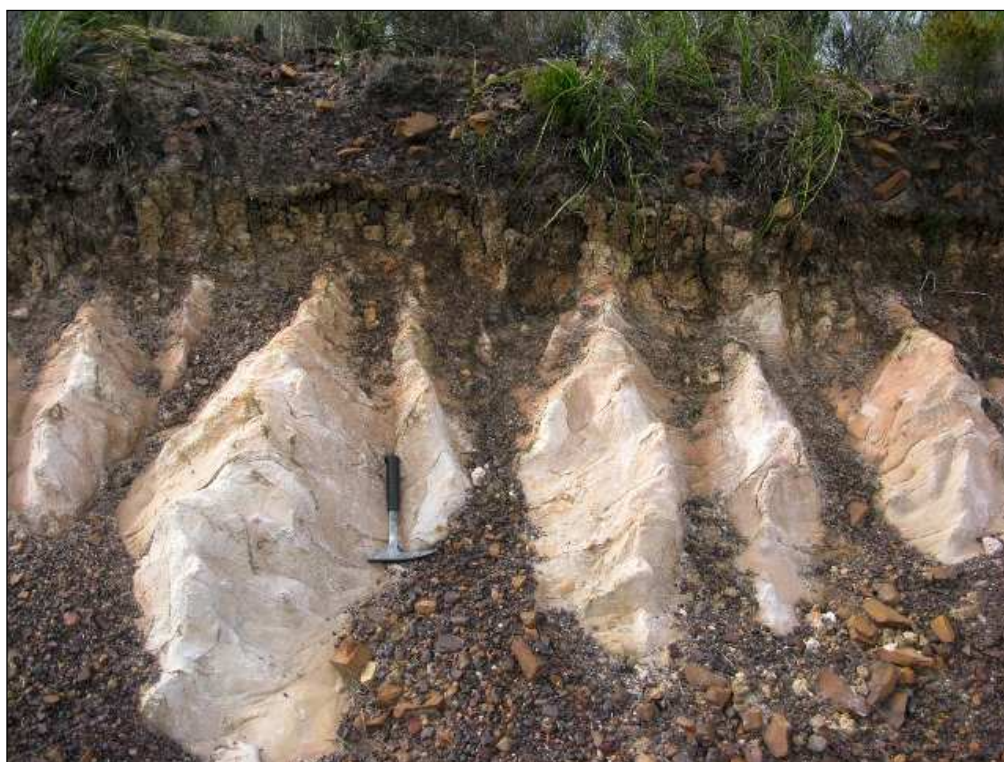
Fig. 9. Cream-coloured, deeply weathered claystones overlain by gravelly soil, R62 road cutting near the Jumanji Nature Reserve (Hammer = 27 cm) (Loc. 039).
