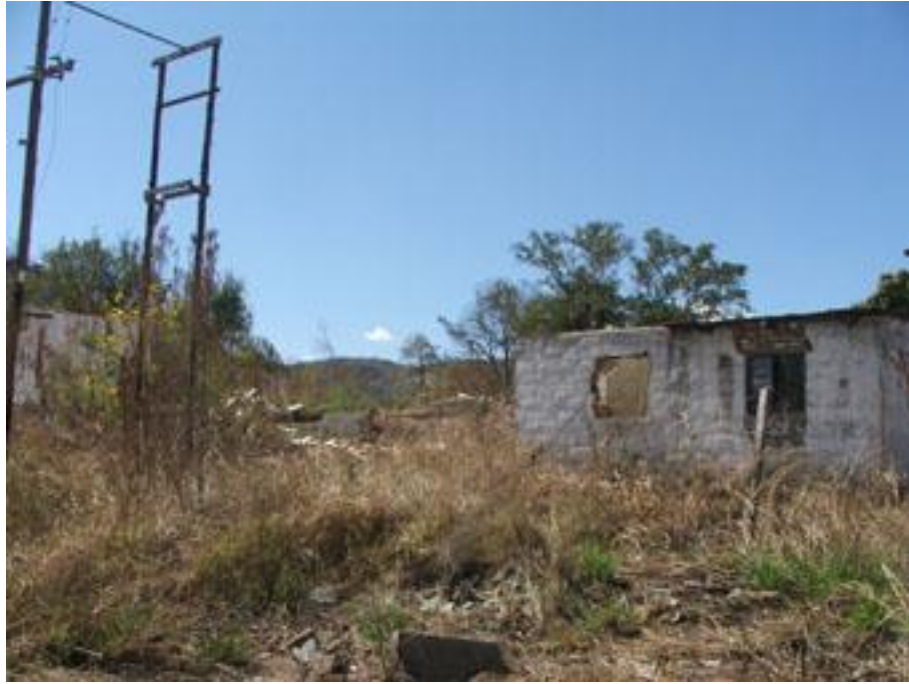
Figure 16. Ruins located at Site 14, photo taken in eastern direction.
