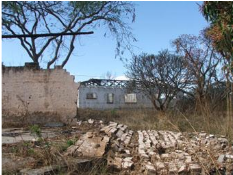
Figure 17. Ruins located at Site 14. Photo taken in eastern direction.
