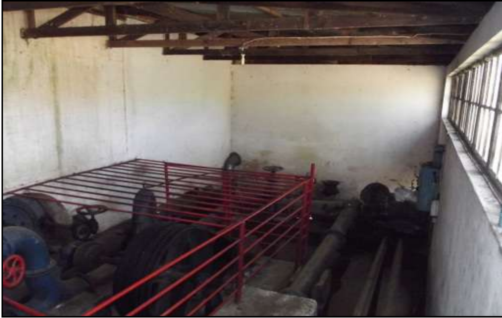
Fig. 11. Site KH 7. Inside the turbine building.
