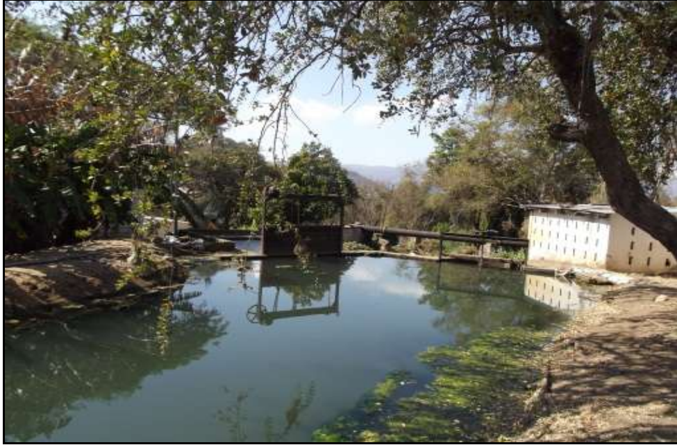
Fig. 9. Site KH 6. This is the location where the 13 foot furrow ends and also where the turbine is located.
