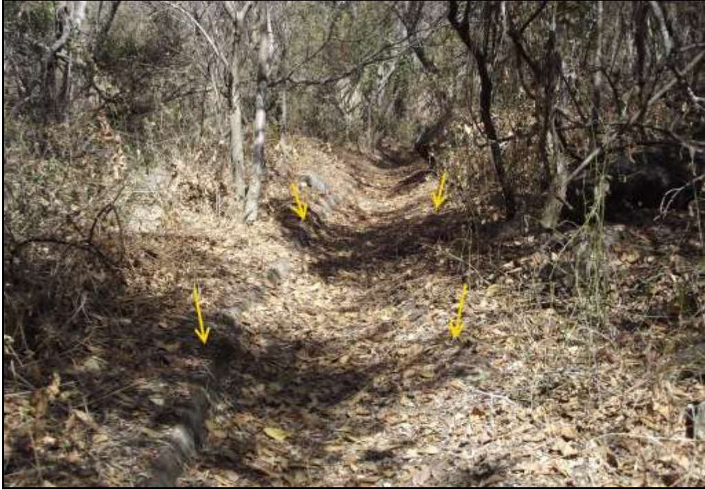
Fig. 13. Site KH 8. The 5 foot water furrow, arrows indicate its concrete sides.
