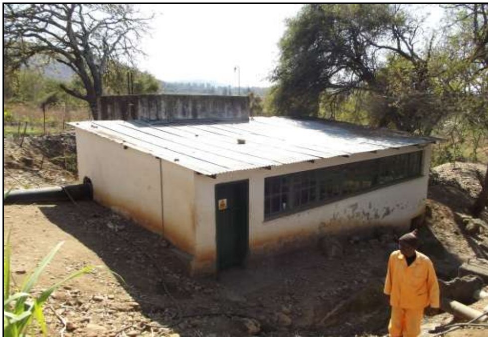
Fig. 10. Site KH 7. The building in which the current turbine is located.
