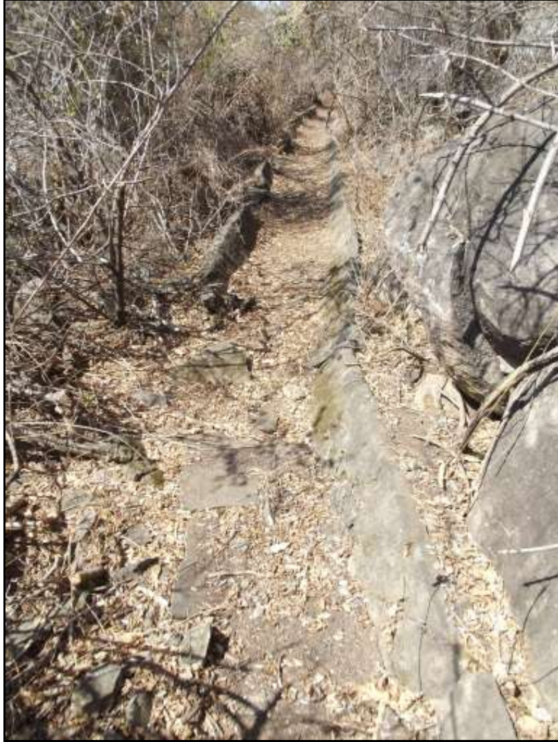
Fig. 15. Site KH 12. Another section where the furrow is damaged.
