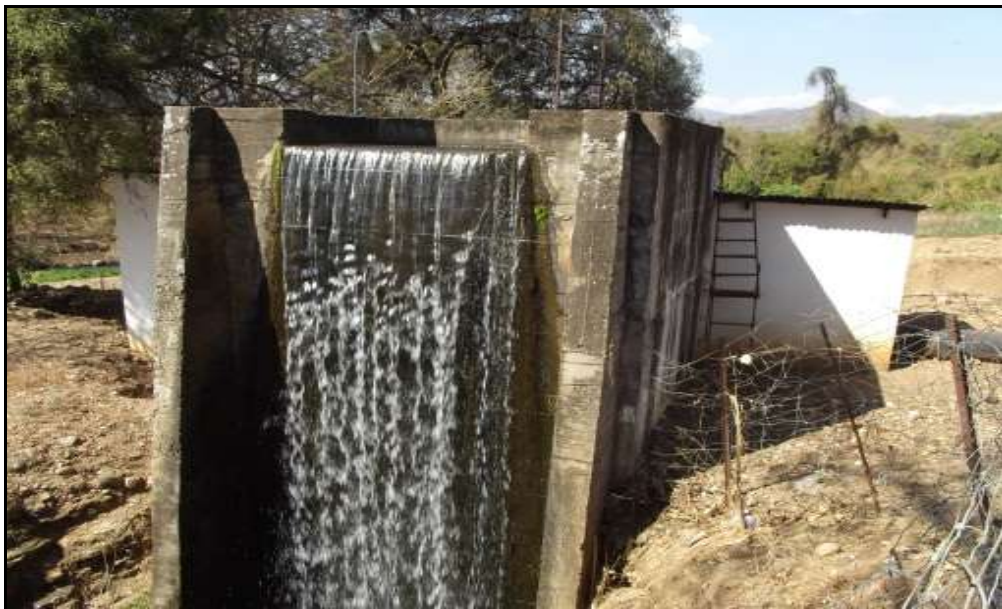
Fig. 12. Site KH 7. The Western side of the turbine building.
