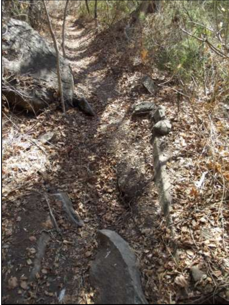
Fig. 14. Site KH 9. A section of the 5 foot wide furrow where it is currently damaged.
