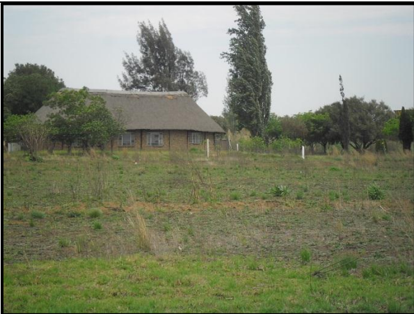
Figure 5: Modern dwelling next to the existing servitude indicated by white markers.
