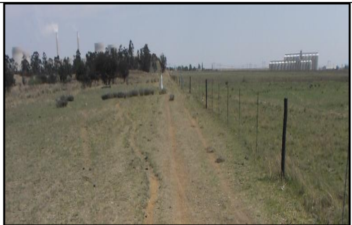
Figure 8: General conditions in the servitude.
