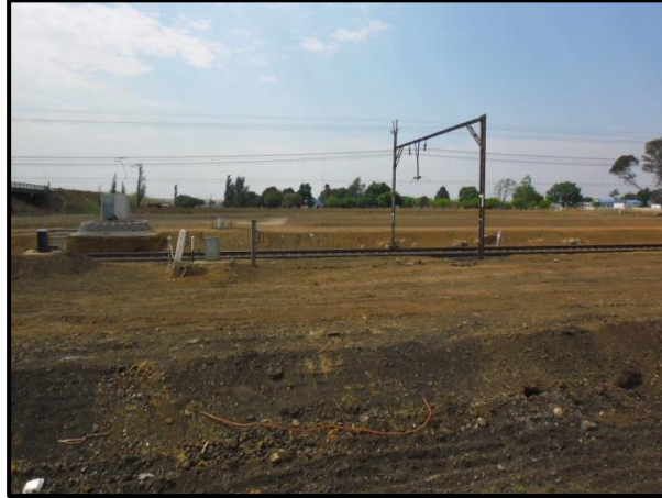
Figure 10: Southern view of railway line.
