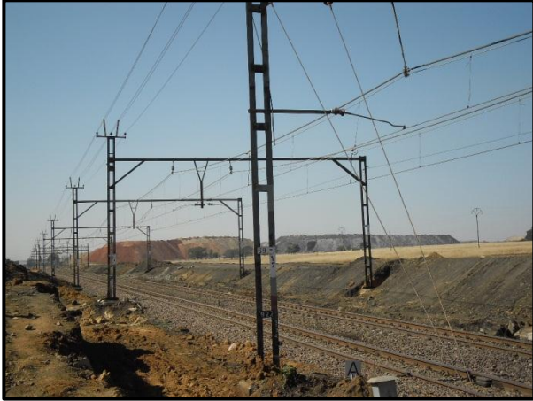
Figure 9: Railway line viewed from the west.
