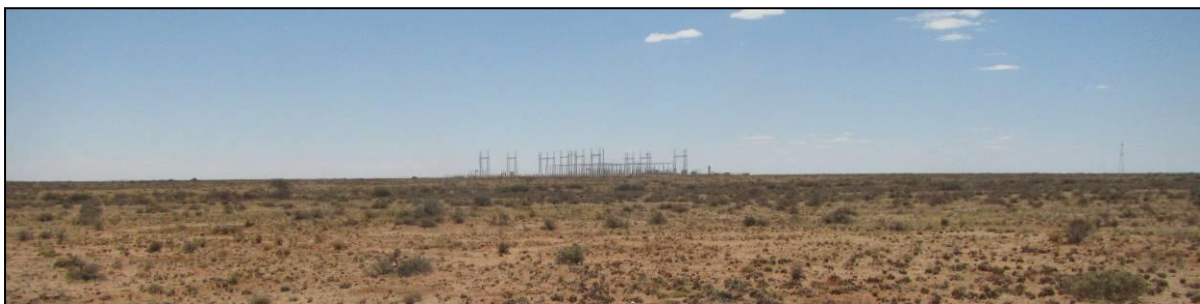
Figure 3: View towards the northeast (from the PV 1 site just north of the railway line) of the Nieuwehoop Substation currently under construction.
