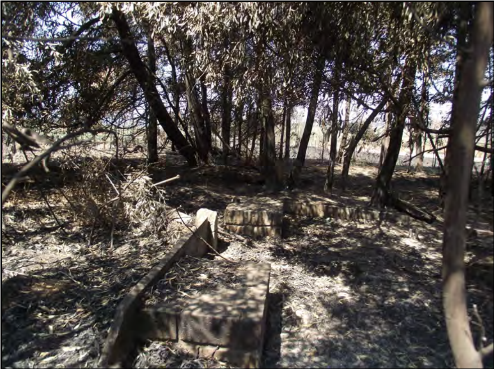
Fig. 9. Site WK 5. Small retaining walls.
