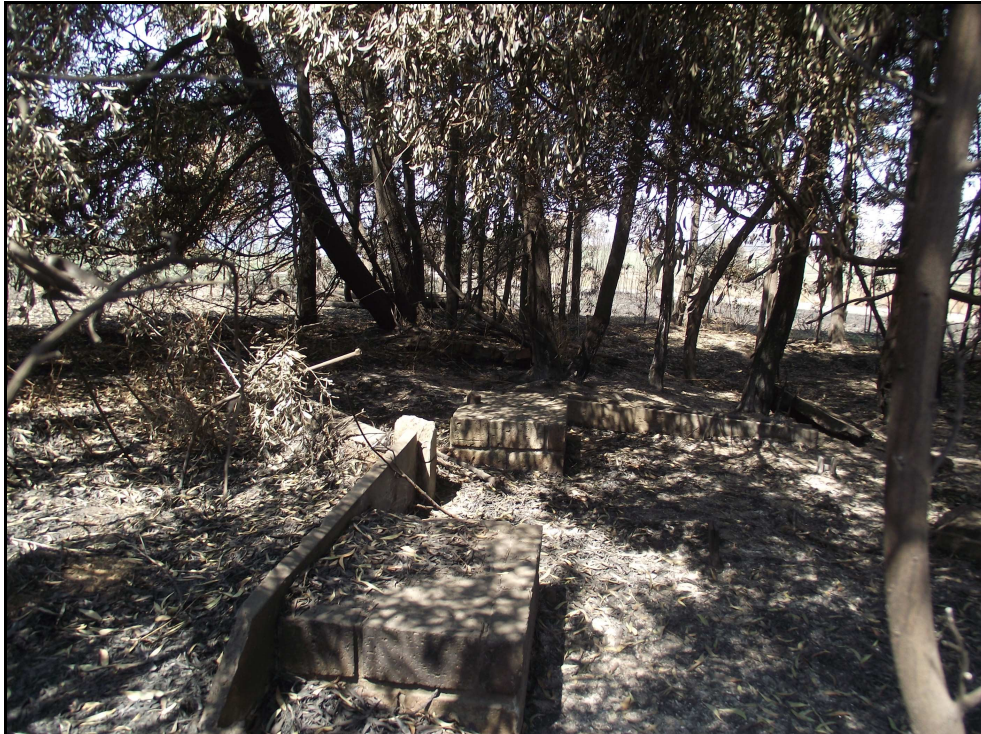
Fig. 9. Site WK 5. Small retaining walls.
