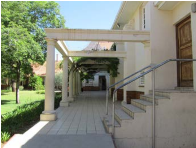
Figure 58: Pergola to the east of the school hall.
