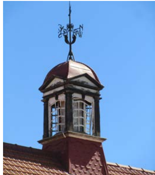
Figure 69: Lantern on the main roof
