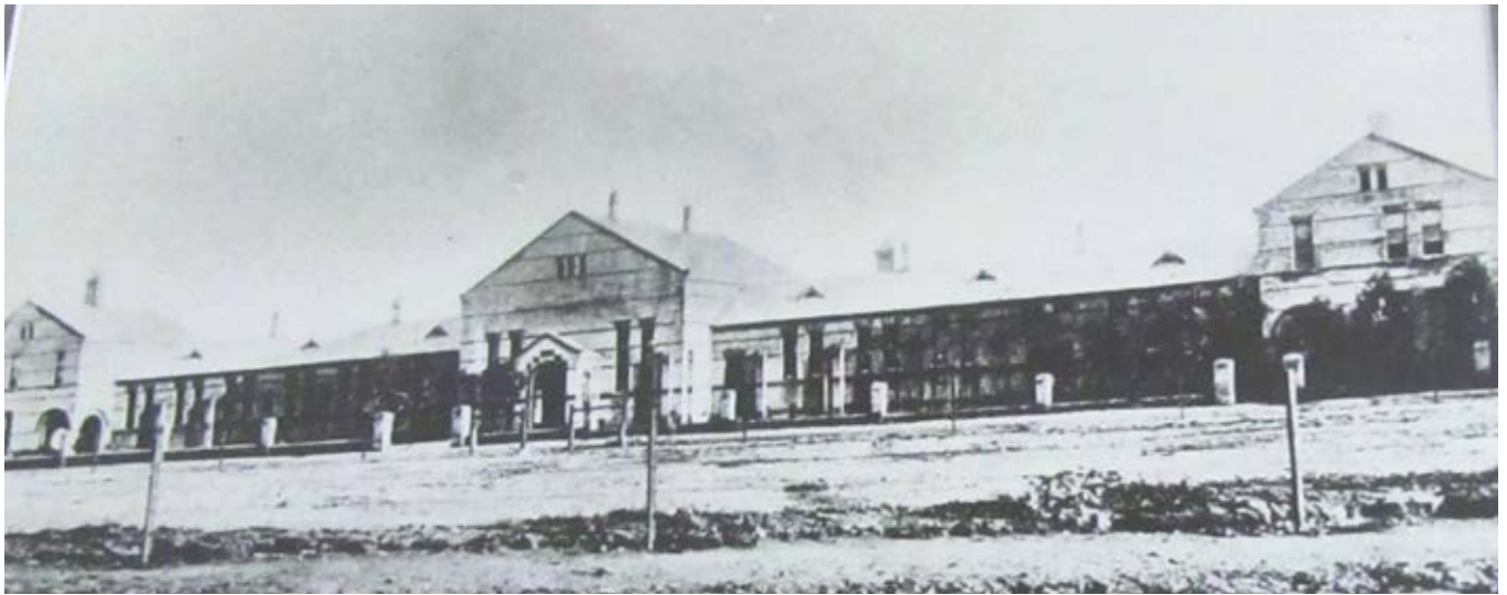
Figure 6: The original 1888 Boys High School Buildings (Kimberley Boys High School Archive)
