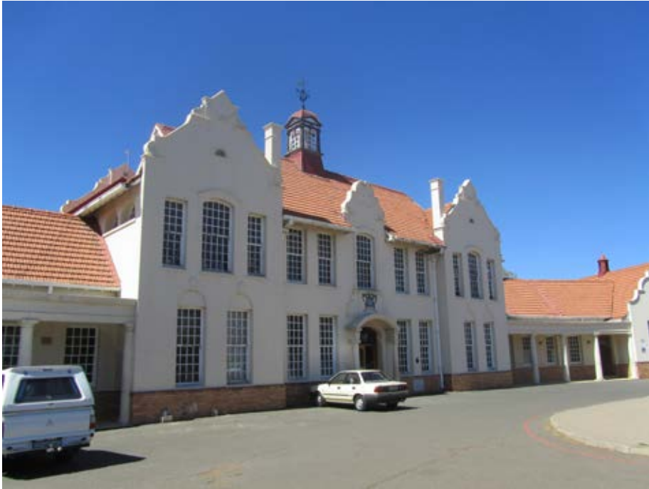
Figure 40: central portion of main facade
