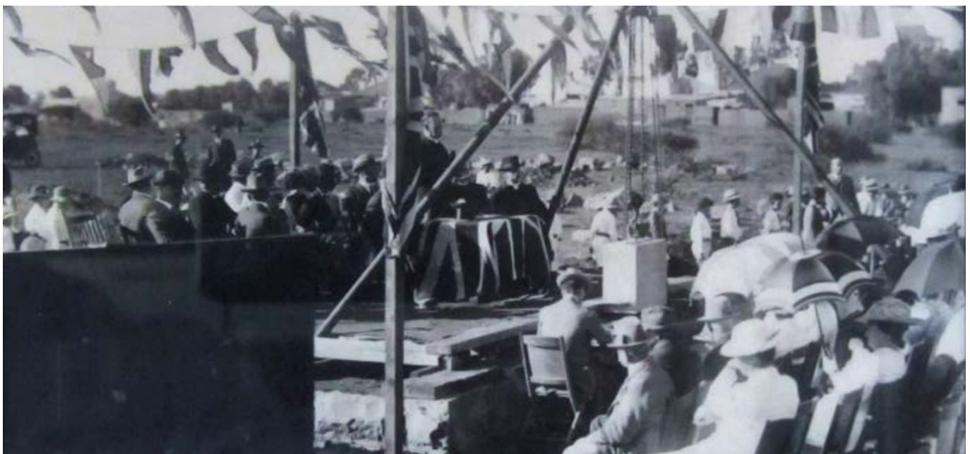
Figure 7: The laying of the foundation stone for the new school building in 1913 (Kimberley Boys High School Archive)
