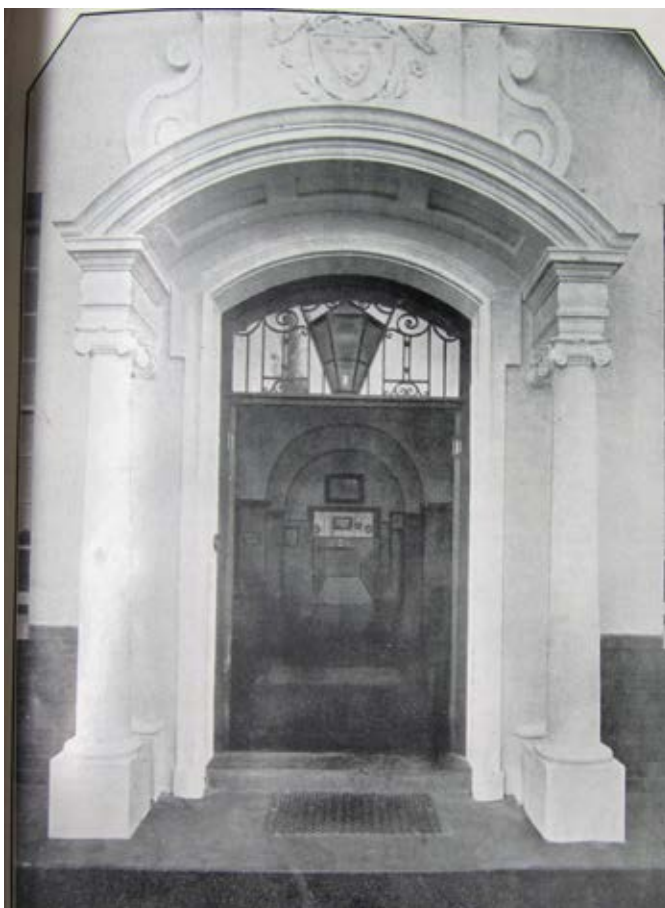
Figure 10: The main entrance looking towards the hall (Kimberley Boys High School Archive)
