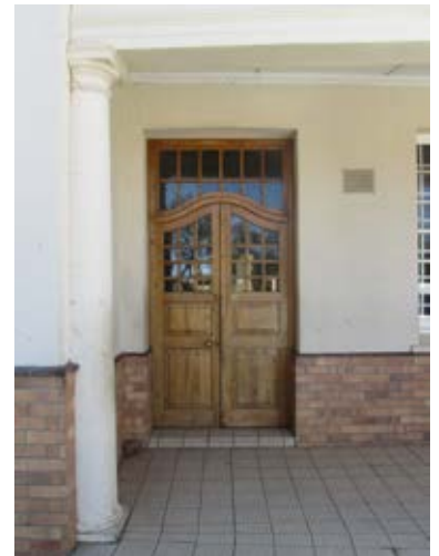
Figure 41: Side door of west wing
